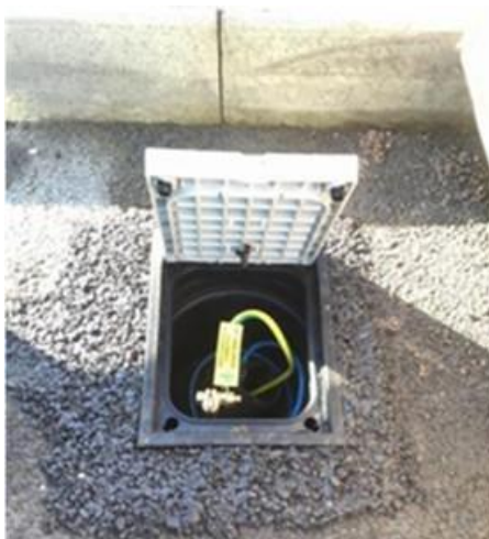
FIGURE 3: LOCALIZED TT EARTH SPIKE
