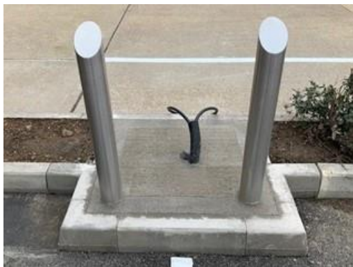
FIGURE 5: STAINLESS STEEL PROTECTION POSTS
