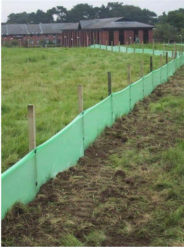
Example of protective newt screed.
