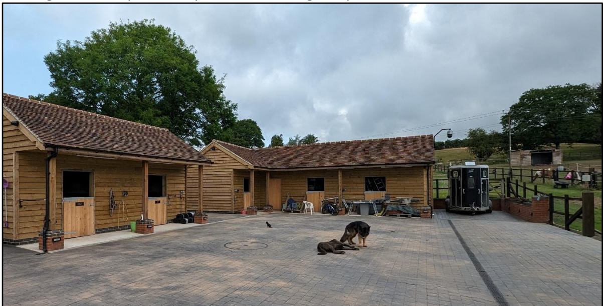
Figure 2: The Stable Buildings Permitted by Planning Application Ref 21975 Under Construction showing increase in permitted yard area to the right of photo
