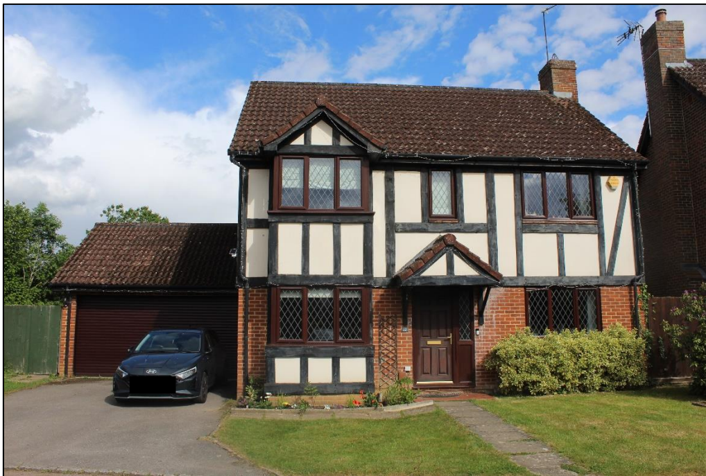
Photograph 1 – Front elevation as viewed from Woodward Close
