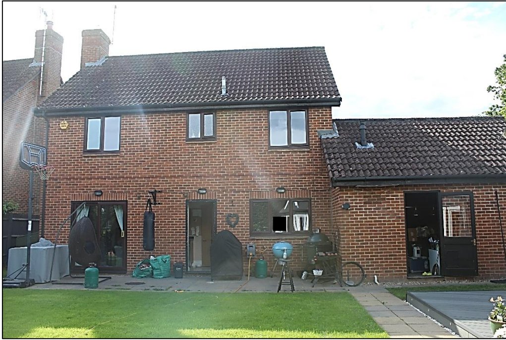
Photograph 2 – Rear view of the property as viewed from the garden
