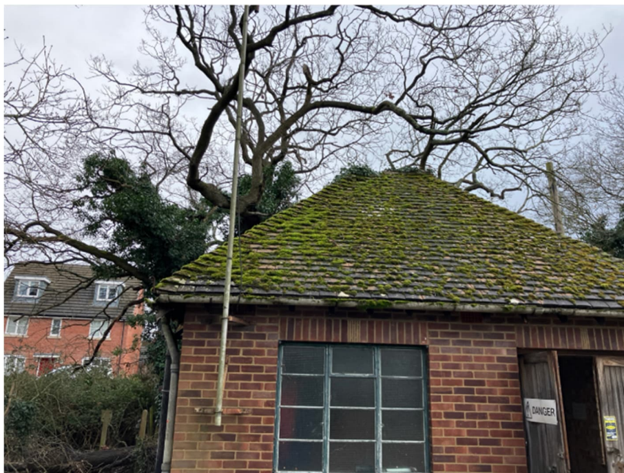
Plate 2. Building 1, looking east
