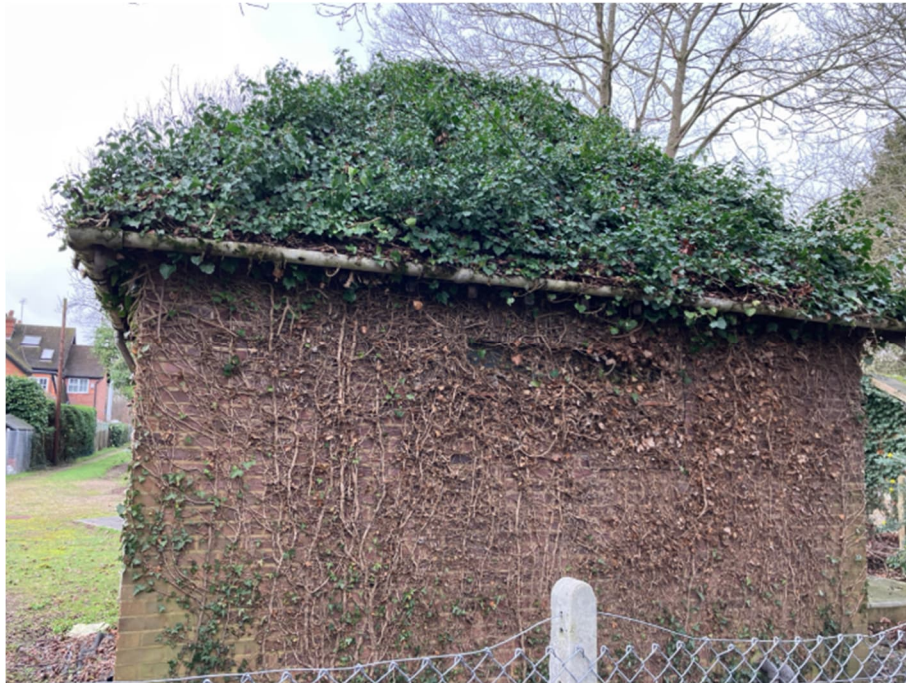
Plate 1. Building 1, looking west
