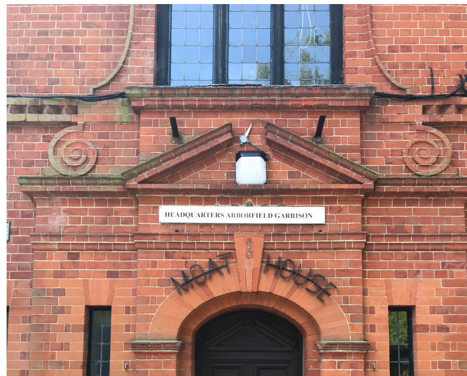
Figure 3.11 Moat House Primary Entrance (Site Visit July 2024)
