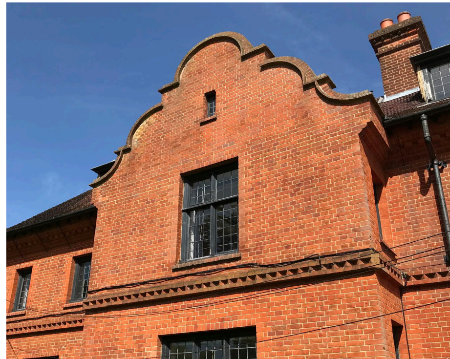
Figure 3.9 Moat House Shaped Gable (Site Visit July 2024)
