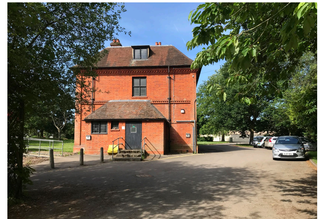
Figure 3.12 Moat House East Elevation (Site Visit July 2024)
