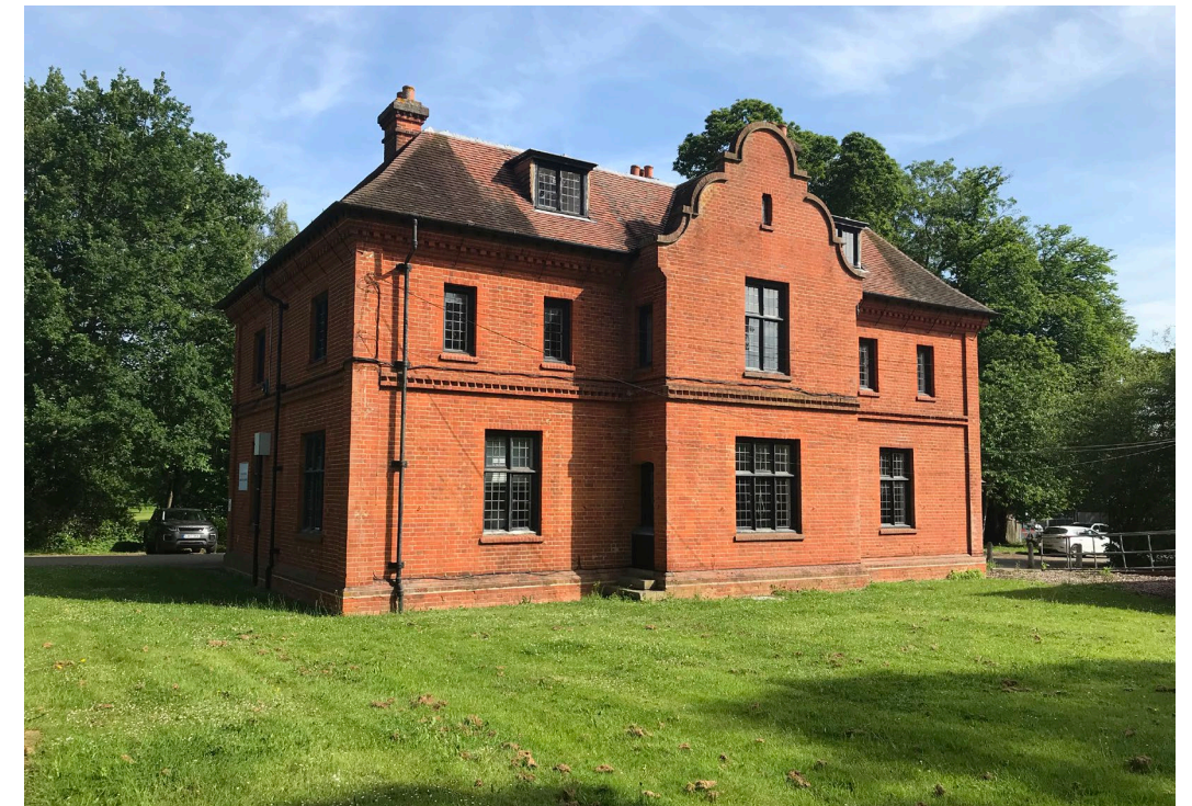
Figure 3.10 Moat House South Elevation (Site Visit July 2024)
