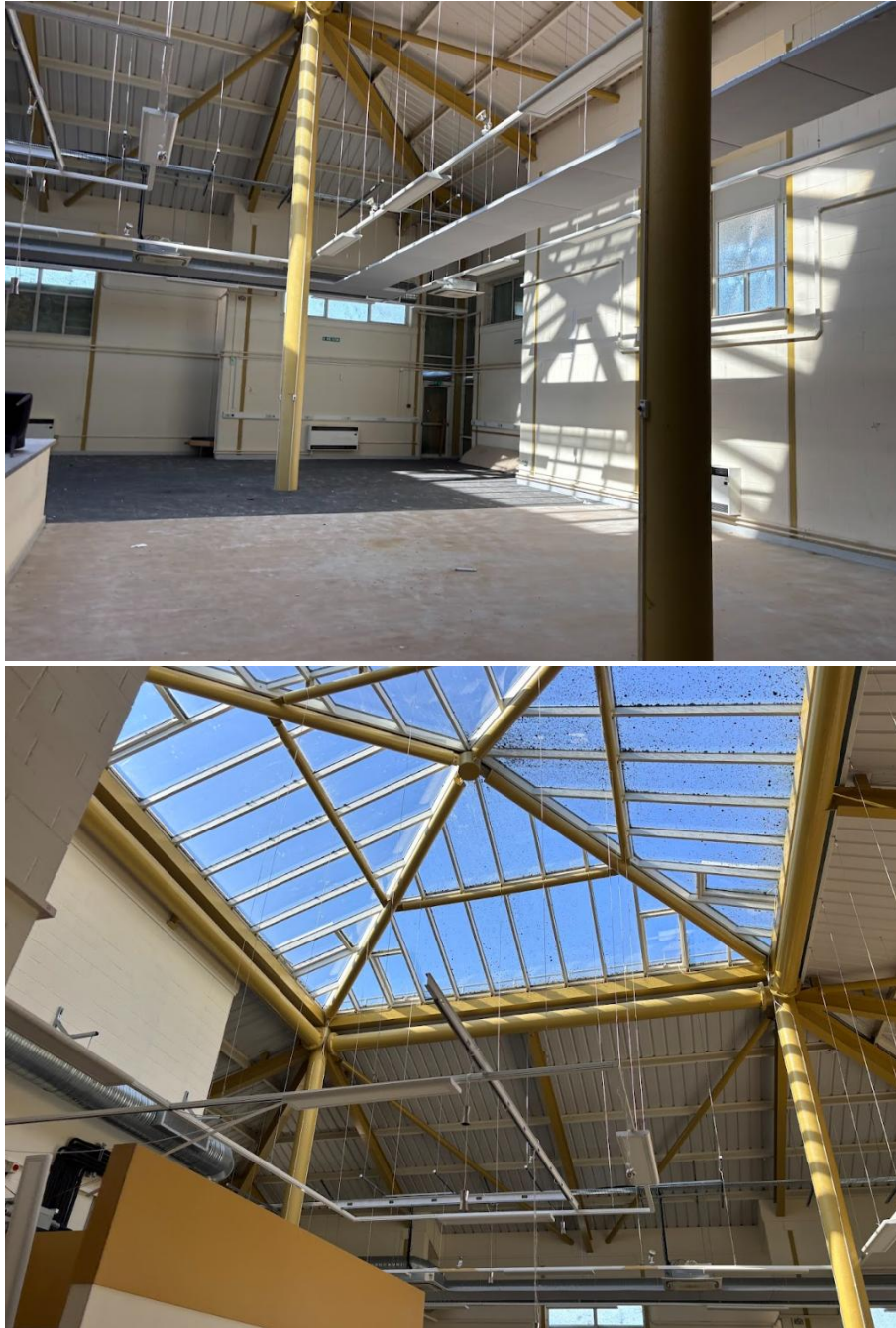
Figure 7. Internal aspect of the building NW16 (taken March, 2026).
