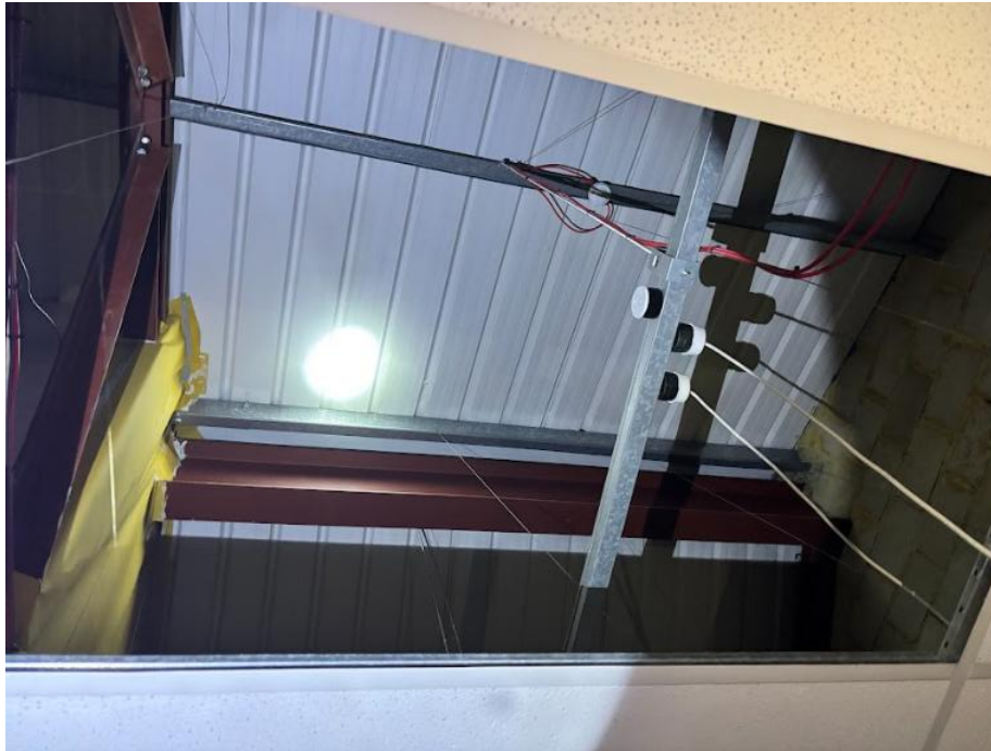
Figure 8. Internal false ceiling aspect of the building NW16 (taken March, 2026).
