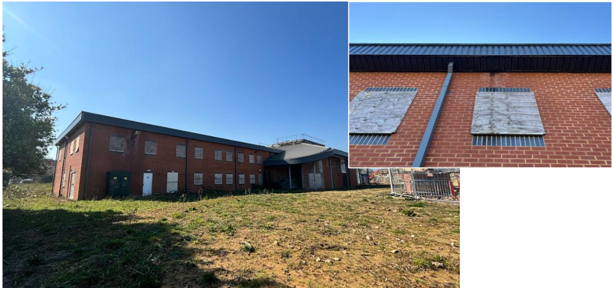
Figure 6. North-eastern elevation of building NW16 showing a close up of the tightly sealed structure (taken March, 2026).
