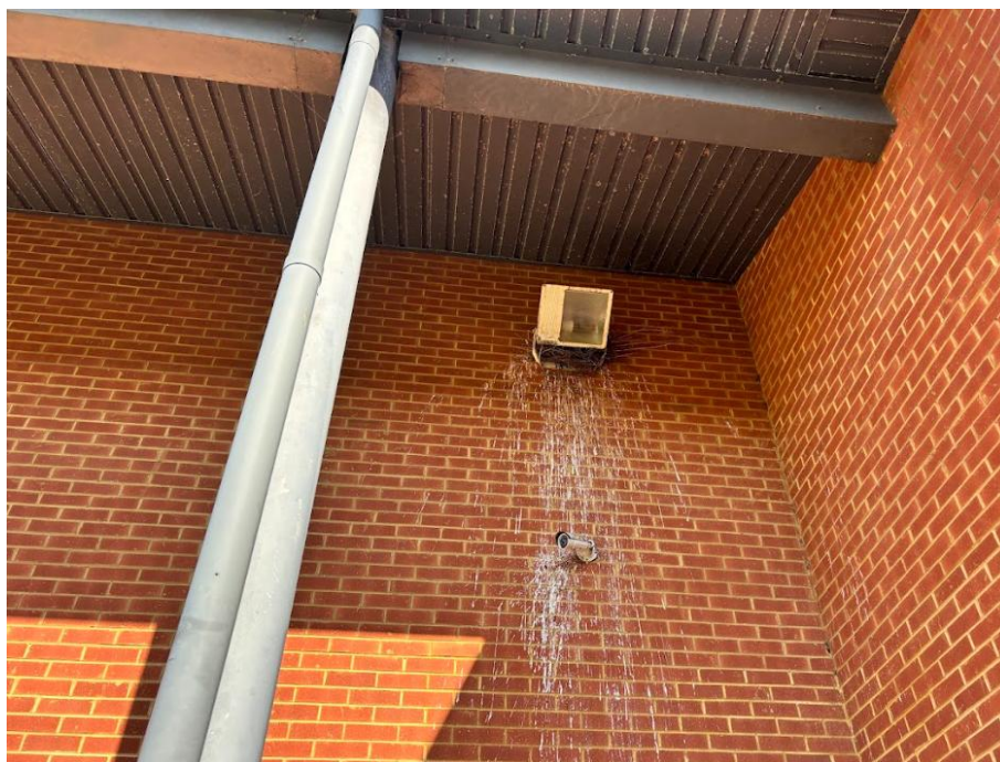
Figure 13. A disused birds nest identified on the southern elevation of building NW16 (taken March, 2026).
