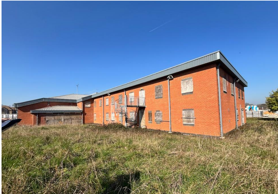
Figure 5. South-eastern elevation of building NW16 (taken March, 2026).
