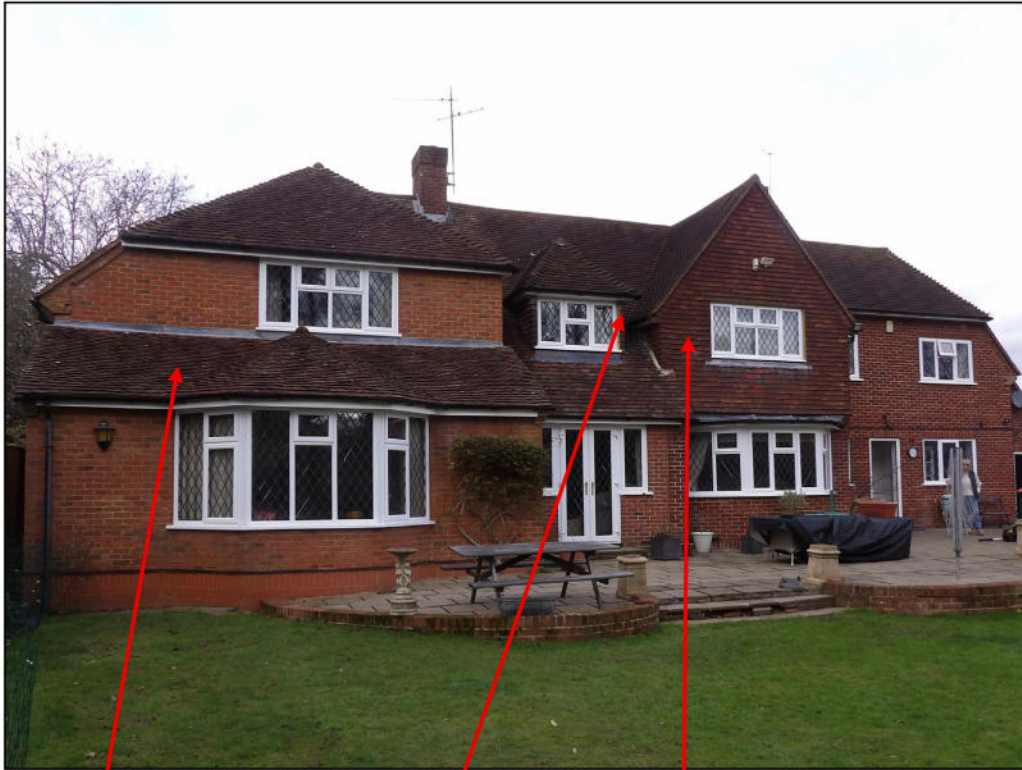
Rear of property emergences
