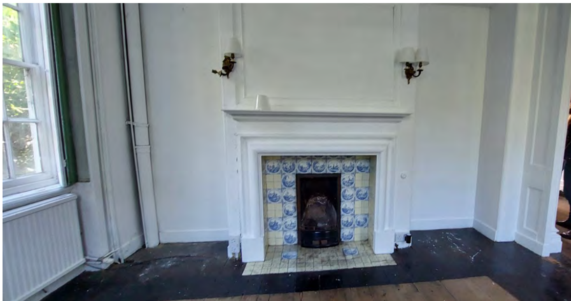
Internal soil stack in room to left of historic tiled fireplace
