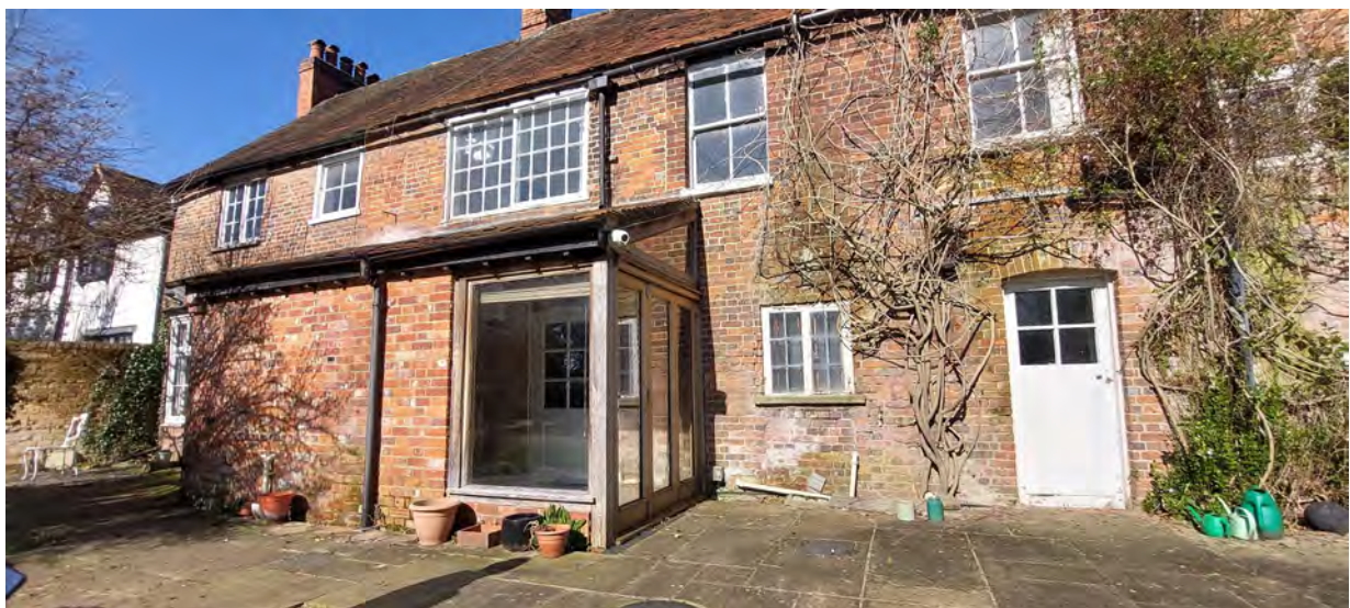
Bay window at Rose Cottage and western side of lean-to extension
