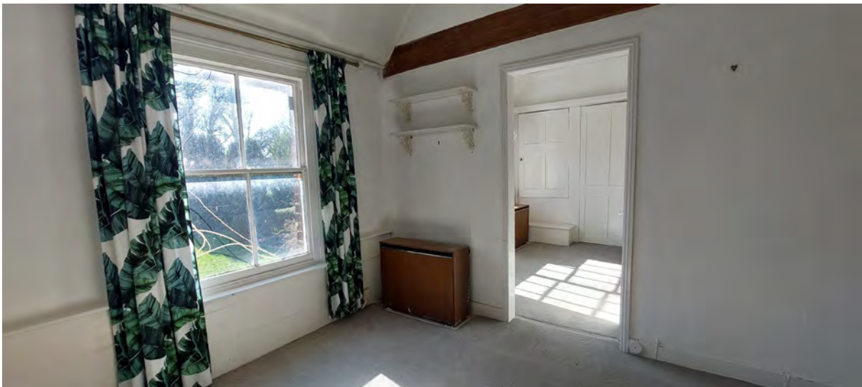
Beams and partition wall on first floor
