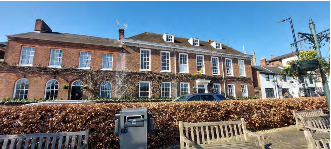
The Grade II listed The Coach House and Rectory
