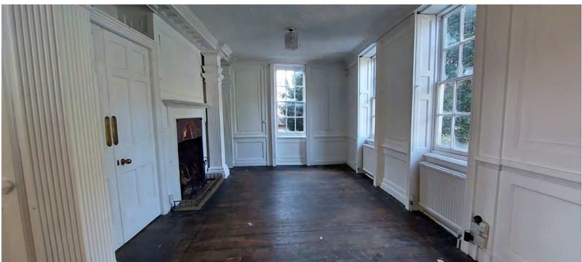
Historic panelling, cornicing, skirting, columns, fireplace in room to right side of ground floor entrance hall
