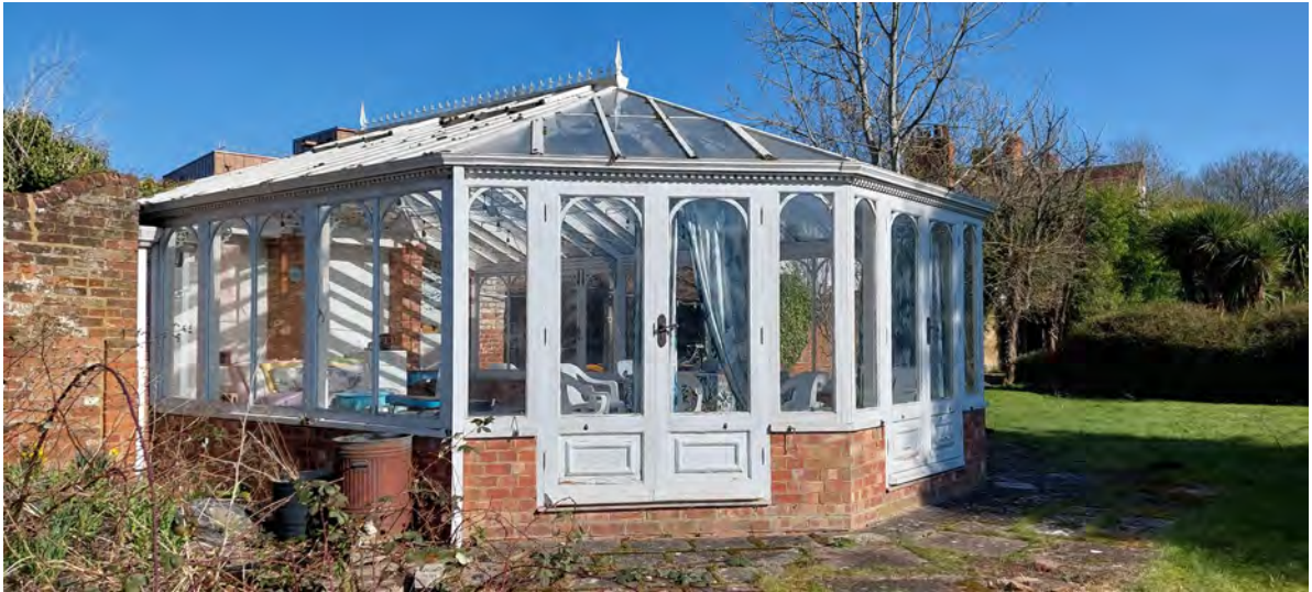
Conservatory with new apartment block rising behind and Site in background to right
