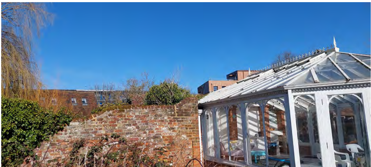
Historic brick boundary wall and conservatory with new apartment block rising behind
