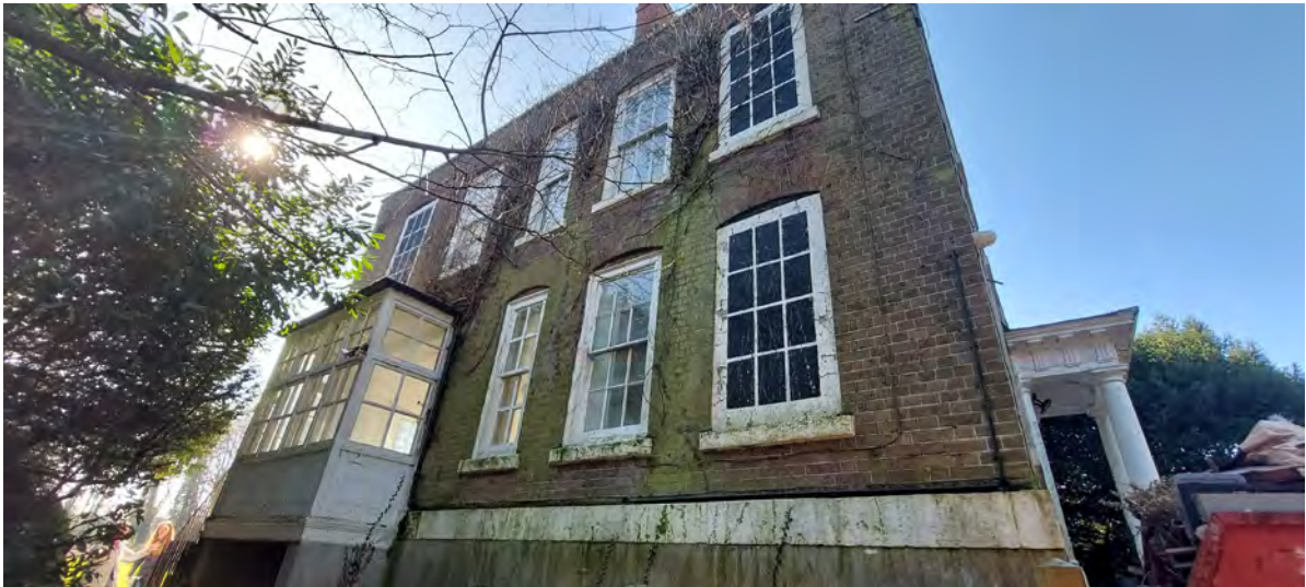
Eastern elevation with blind windows
