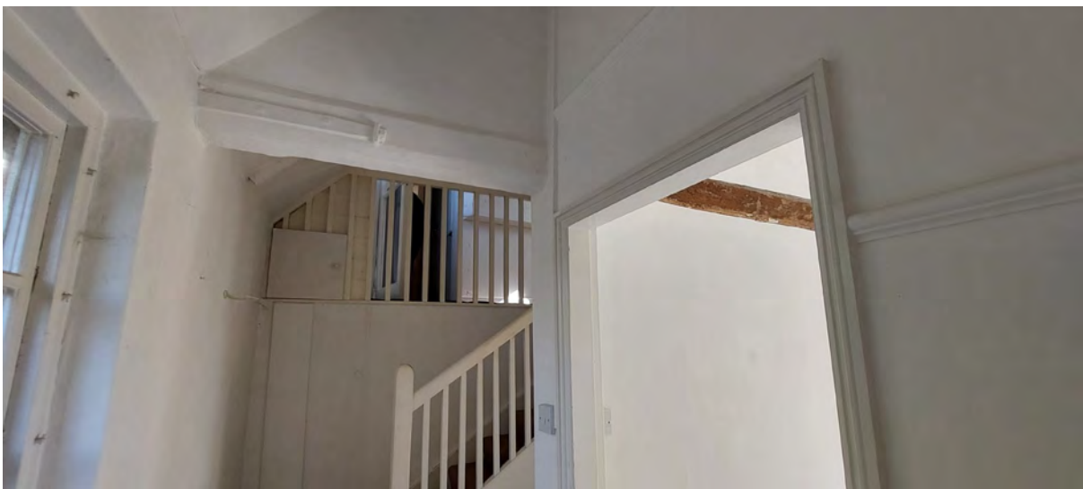
Beams on first floor of Rose Cottage
