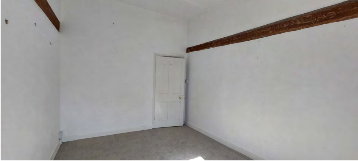
Historic beams on first floor
