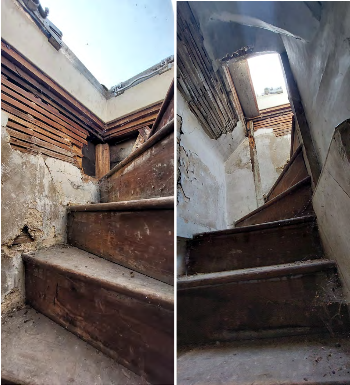
Stairs to roof
