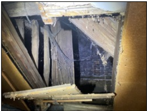
Figure 23 – Roof void 4 inside south-western roof pitch.
