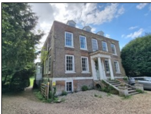
Figure 17 – North-eastern corner of the main house.
