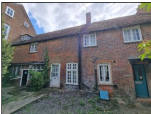
Figure 29 – Northern elevation of Rose Cottage.
