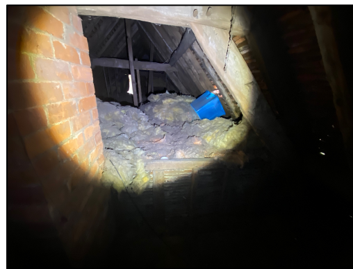
Figure 32 – Interior roof void of the cottage looking east.
