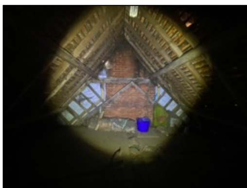
Figure 31 – Interior roof void of the cottage looking west.
