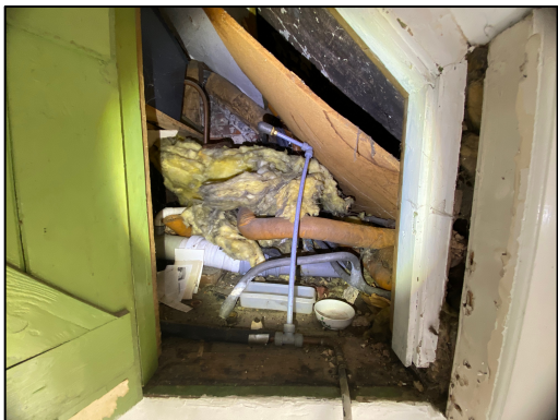
Figure 20 – Roof void 1 in side eaves of the bathroom.
