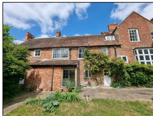
Figure 30 – Northern elevation of Rose Cottage.
