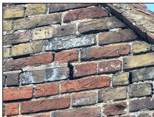
Figure 25 – Southern elevation of the main house.
