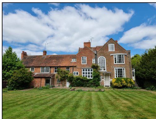
Figure 18 – Southern elevations of the main house and western Rose Cottage.
