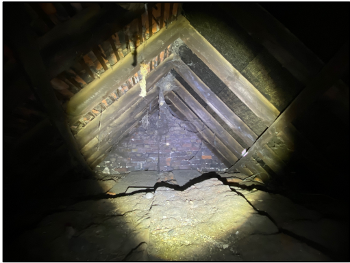
Figure 22 – Roof void 3 inside south-eastern roof pitch.
