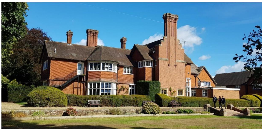
The main entrance front on the North side of Holme Grange.
