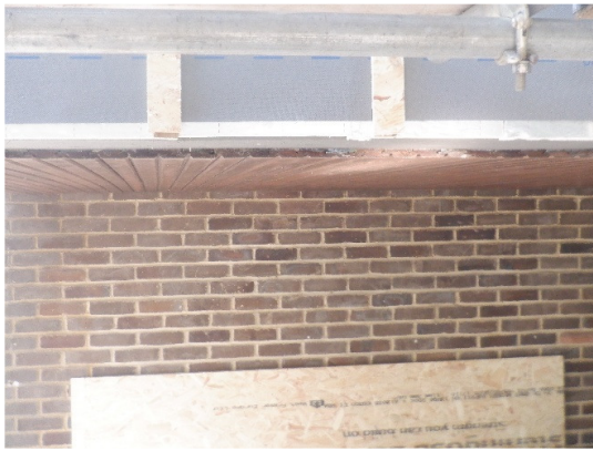
Photograph 8. Roof beneath the front gable end tightly fitted with interlocking timbers.
