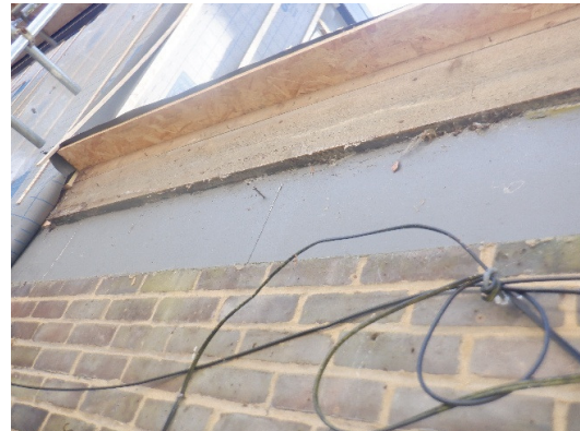
Photograph 4. Concrete beam around the house.
