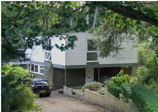
Photograph 5. Former uPVC cladding as shown on google maps from 2023.
