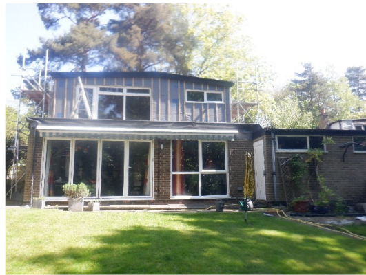
Photograph 2. Rear of the house viewed from the southwest.
