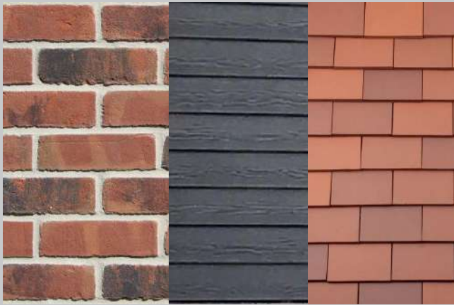
Multi-tonal red brick. Some black weatherboarding, and tile hanging.
