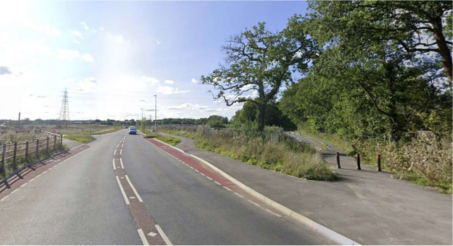
03 View from Nine Mile Ride Extension looking west showing the approach to the sites with Parcel 13 on the right
