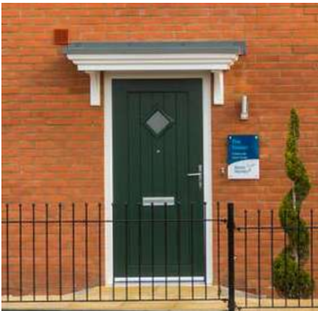
Flat roof canopy
