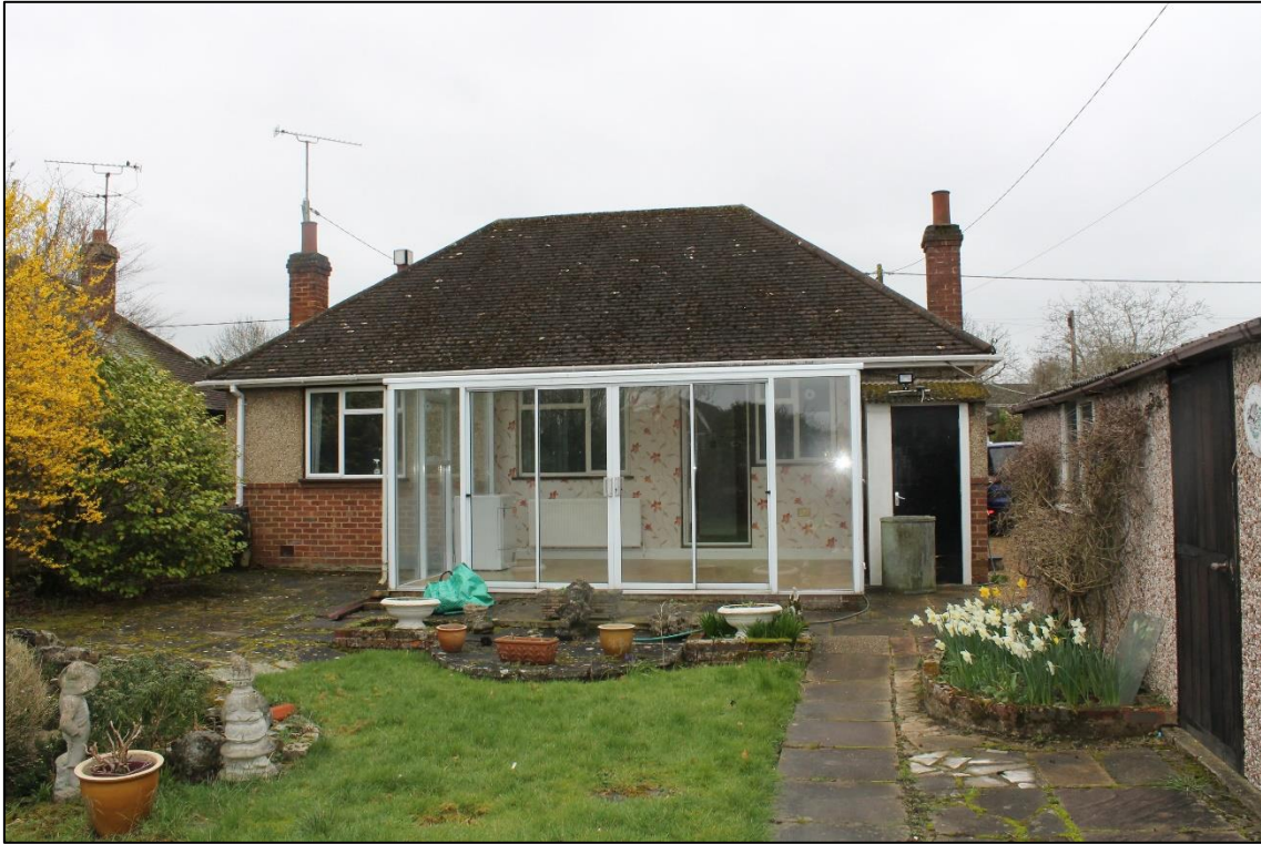
Photograph 2 – Rear elevation as viewed from the garden
