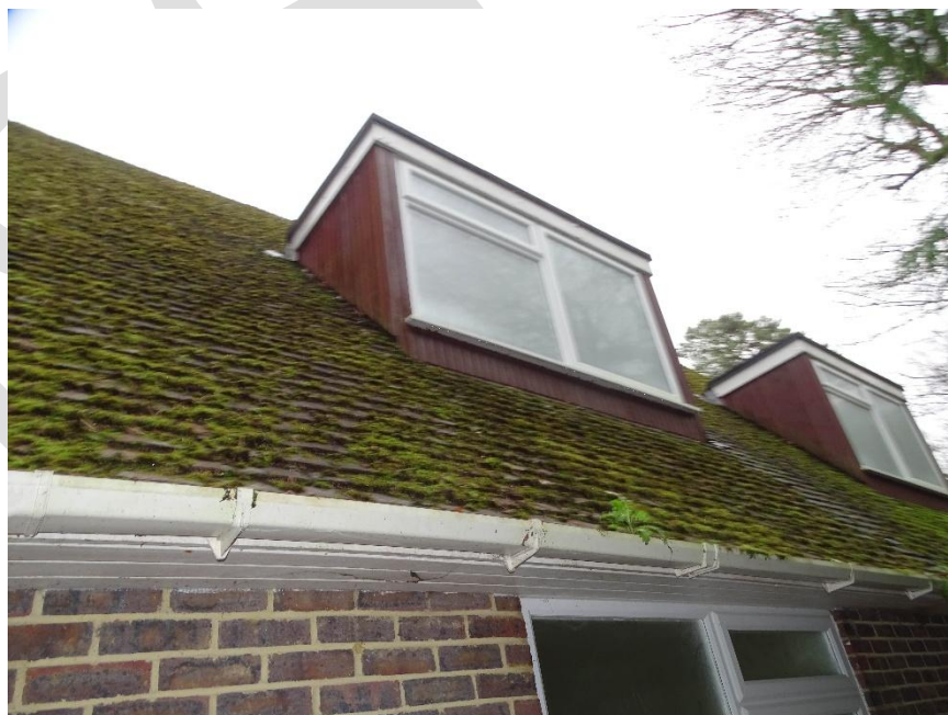
Photo 4: View of ridge, tiles and dormers, east face of property
