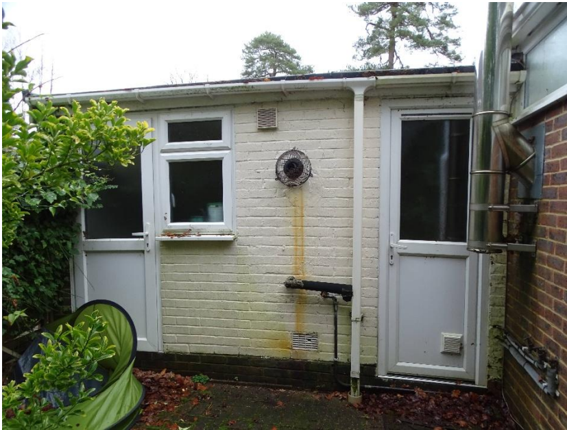
Photo 9: Flat-roofed extension to western side of property
