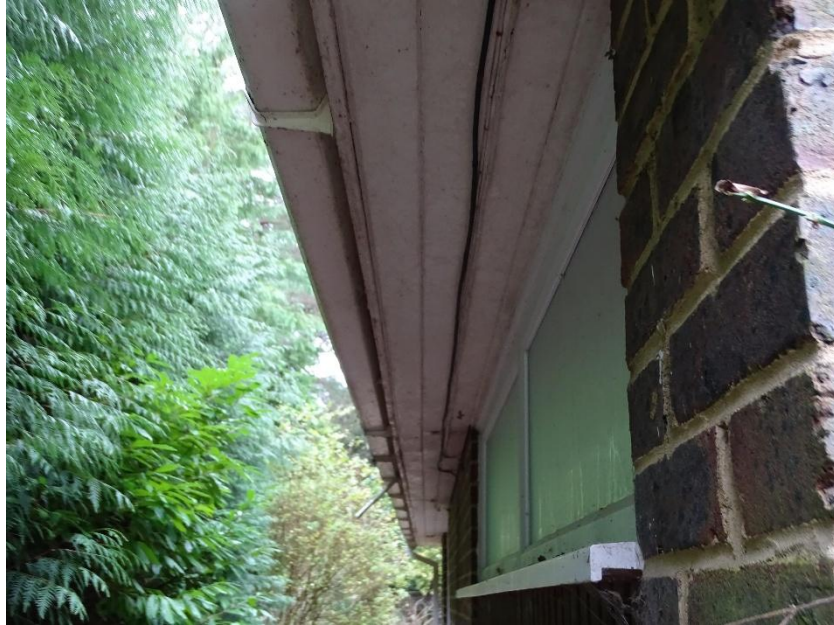
Photo 5: Wooden soffit box along eastern face of property
