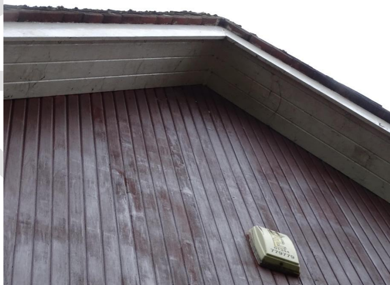
Photo 6: Sealed soffits and wooden cladding at front of property
