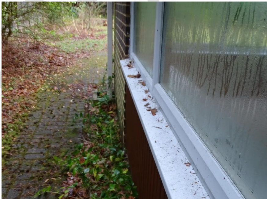
Photo 2: PVC window along west-facing side of the property
