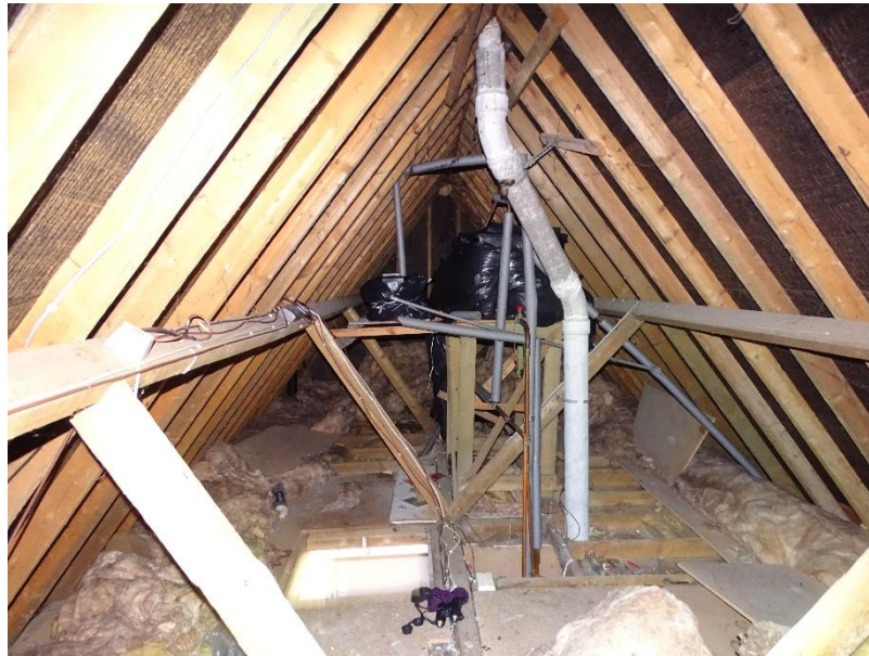
Photo 10: Loft space showing roofing felt onto wooden joists
