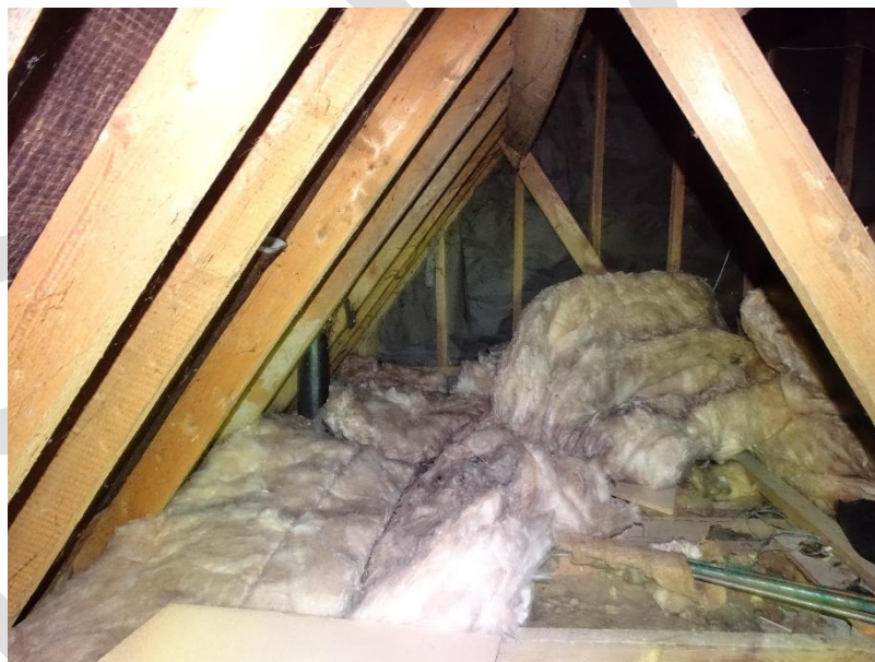
Photo 11: Loft space showing boarding and insulation materials
