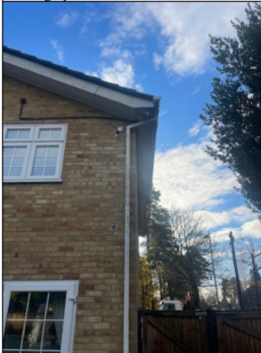
Photograph 7: Soffits in good condition
