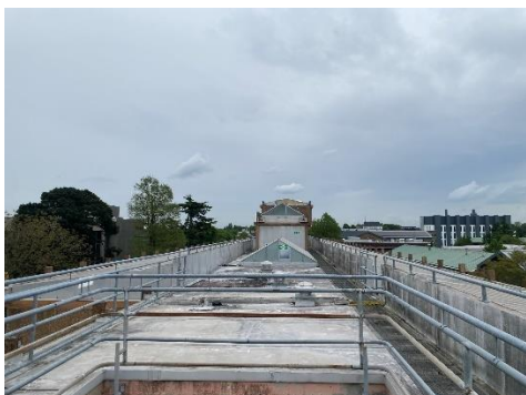
Photograph 45. Level 4 roof (looking east)
