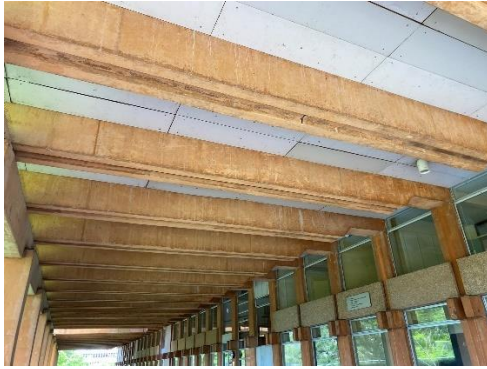
Photograph 13 – Walkway known as Chancellor's Way along North Elevation. The supporting structural columns forming a colonnade
