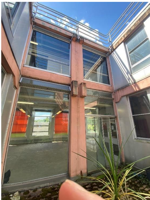
Photograph 31. External light well with non-loadbearing block walls between concrete columns
