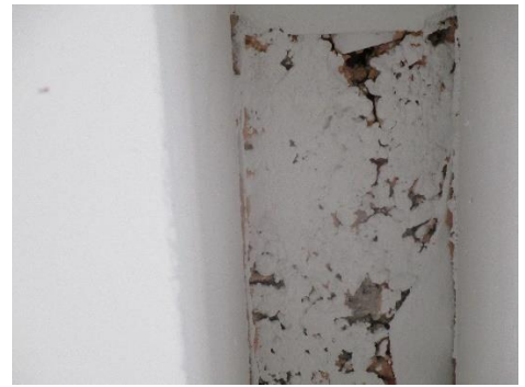
Photograph 44 – Poor compaction and honeycombing issues on slab soffit between PT double beams.
