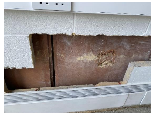
Photograph 24 – 50mm thick concrete block wall forming inner leaf behind precast cladding panels.
