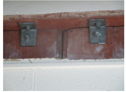
Photograph 22 – Detailed inspection of precast cladding panel fixings at top
