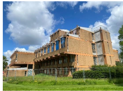
Photograph 4 - South and East Elevations
