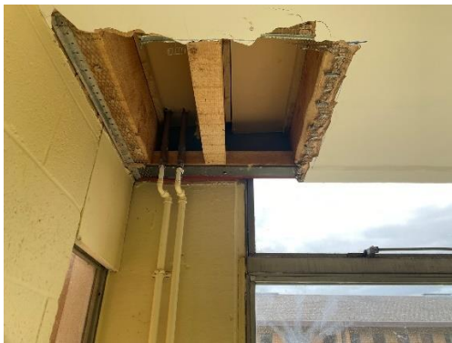
Photograph 39. Timber joists supported on steel beam (PFC) fixed back to existing structure.
