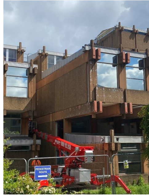
Photograph 2 - Concrete surveys on south elevation
