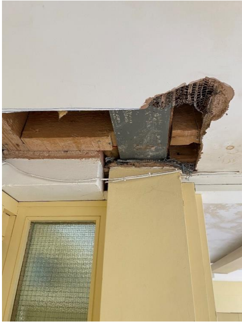
Photograph 37. 1990's Ground floor infill. Steel beam and timber joist floor construction. Supported on new steel columns or Props installed on site.
