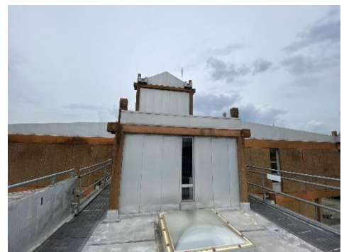
Photograph 46 – Level 4 roof (looking west)
