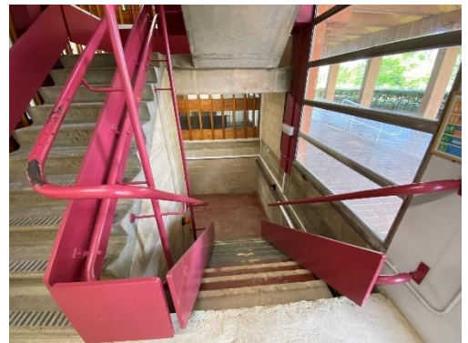
Photograph 40 – East stair core with visual concrete.
