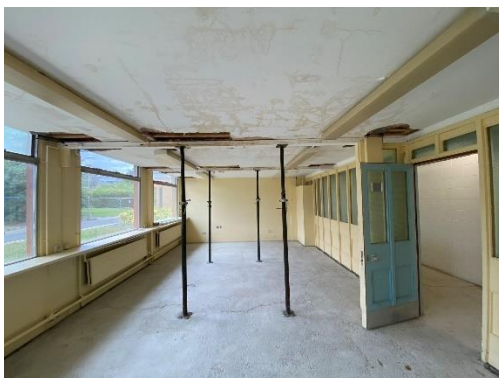
Photograph 35. 1990's Ground floor infill. Props installed on site.
