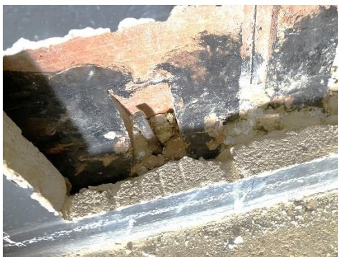
Photograph 23. Detailed inspection of precast cladding panel fixings at base to PT beam below
