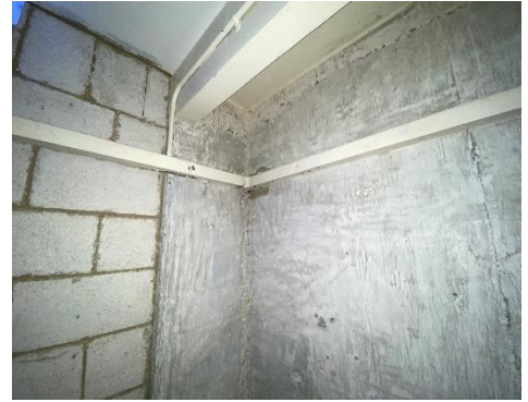
Photograph 28 – Concrete shear wall along north-south direction between columns
