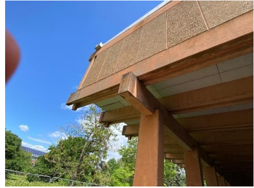
Photograph 14 – Level 2 Transfer beam along north elevation.
