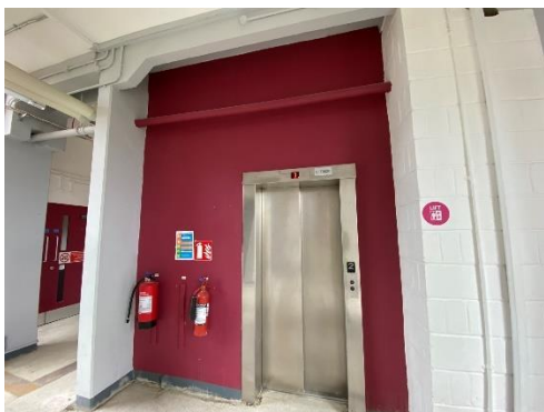
Photograph 29. Concrete shear wall within lift shaft
