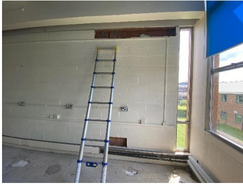
Photograph 21. Internal inspection of precast cladding panel fixings (top and bottom)
