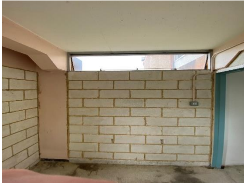
Photograph 27. Non-loadbearing block walls between concrete columns
