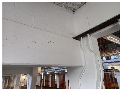
Photograph 30 – Diagonal concrete block wall
