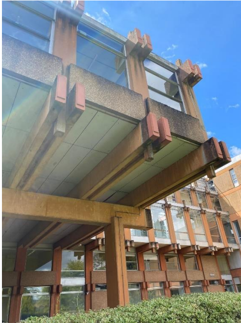
Photograph 5 - South elevation PT beams cantilever
