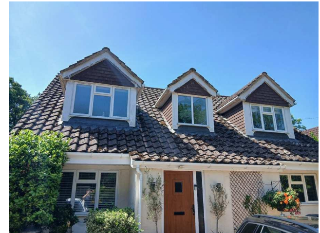
The northern elevation of B1.
