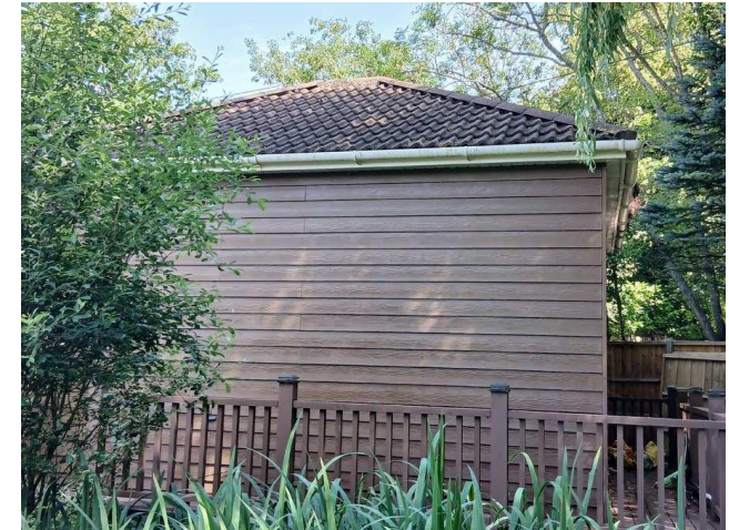
Southern elevation of B3.
