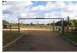
Height-reducing barrier to car park combined with lockable timber access gate and lockable post
