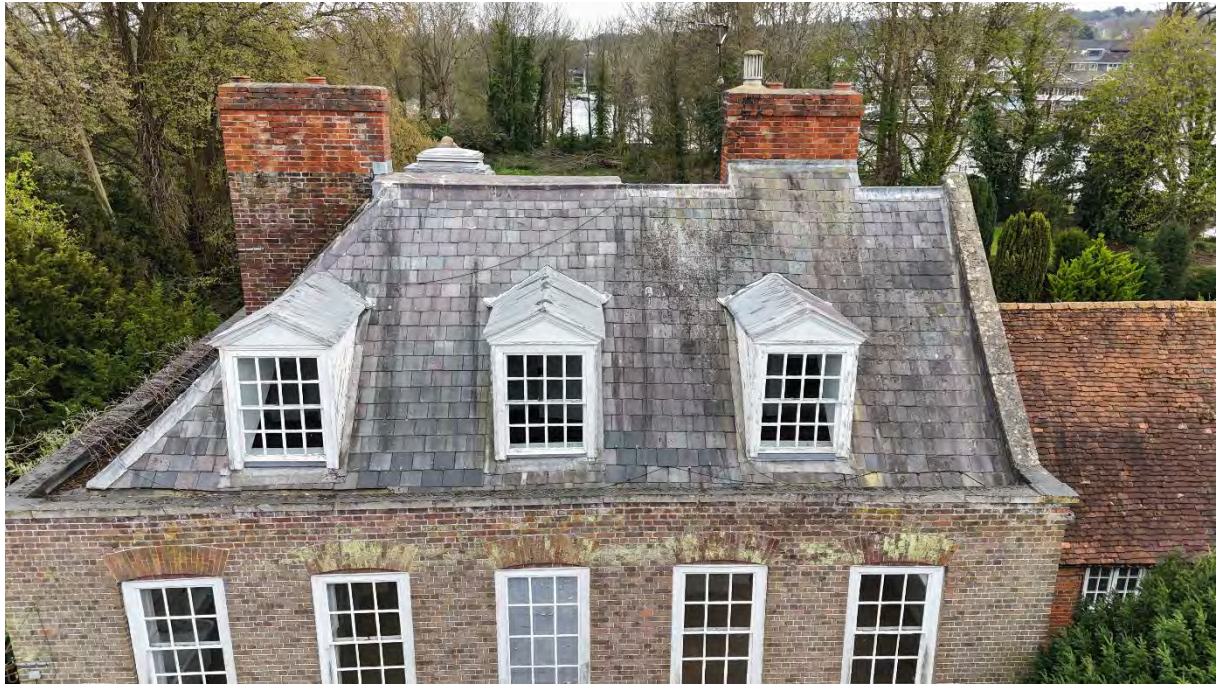
P19 Roof – view front
