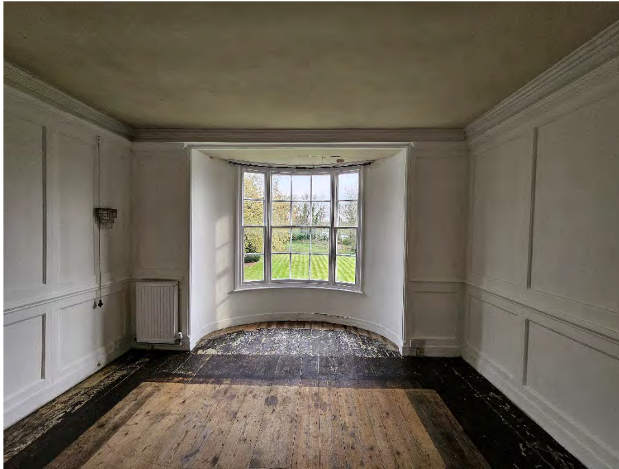
P75 Rear left-hand bedroom – first floor – bay window
