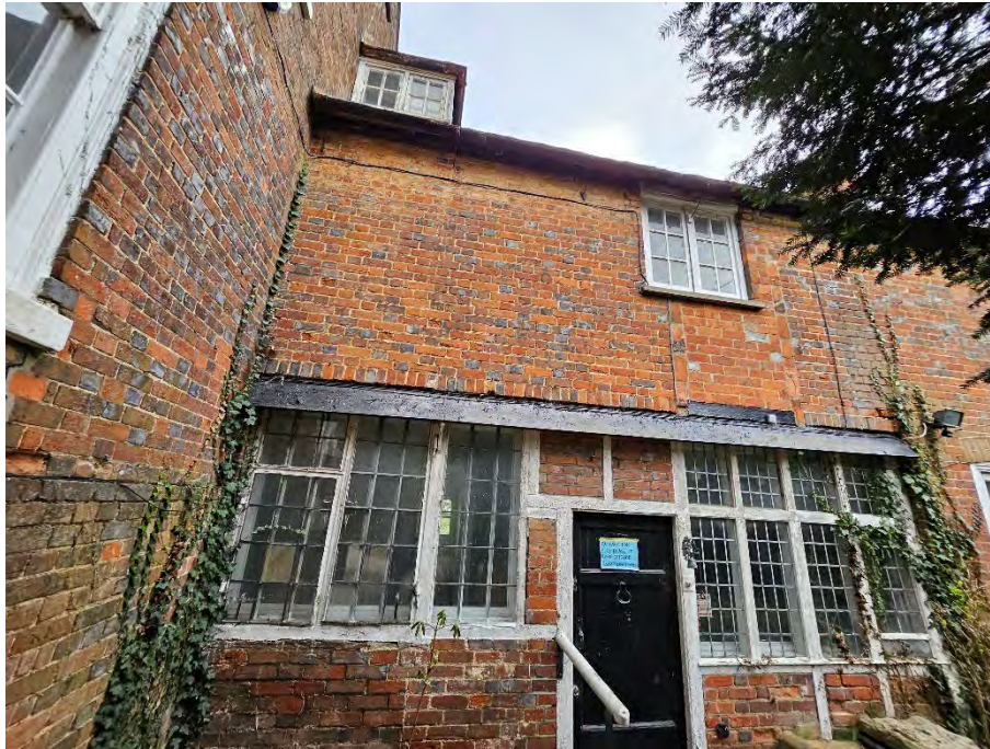
P9 Junction Rose Cottage/Bird Place
