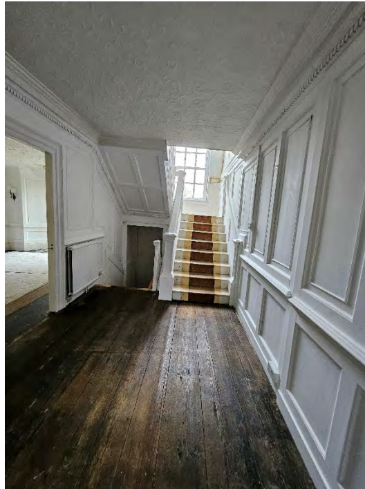
P61 Central hallway – view to rear stairs
