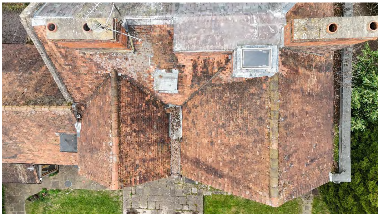
P22 Rear roof
