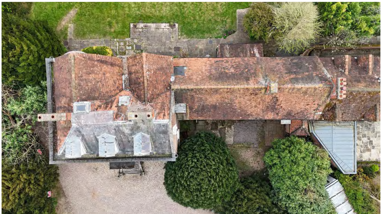
P18 Roof - general
