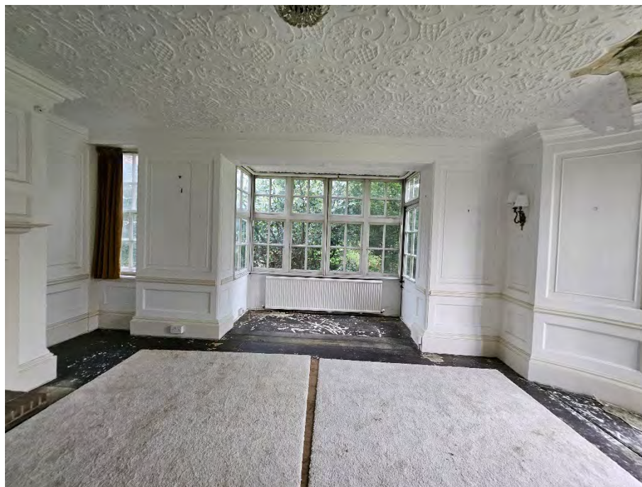
P67 Ground floor – rear left-hand room – view east
