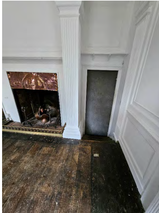
P59 Link access to Rose Cottage – stairs beyond
