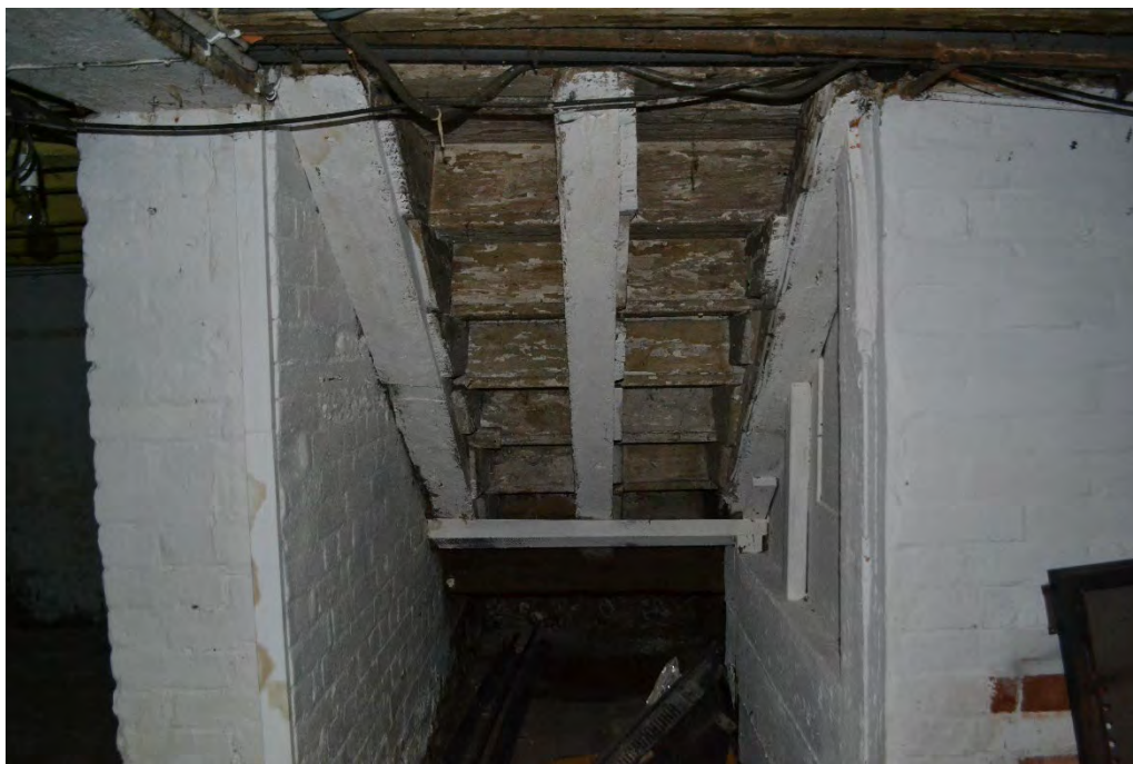
P57 Stairs down from hallway to rear
