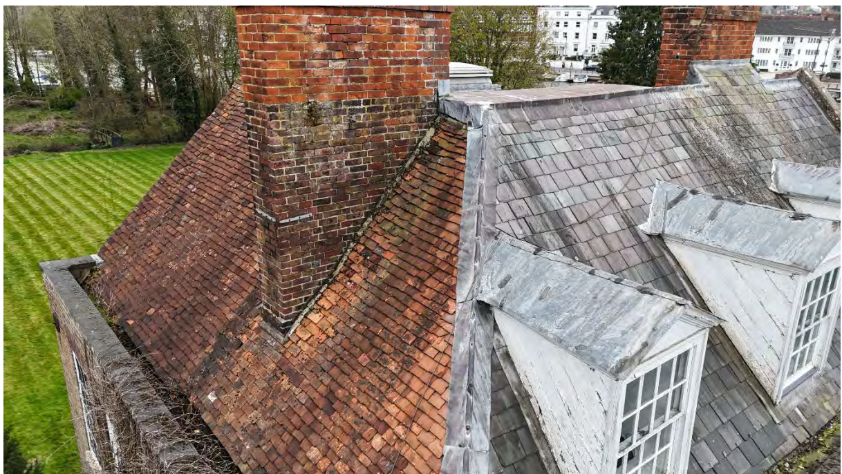
P20 Roof – left-hand elevation
