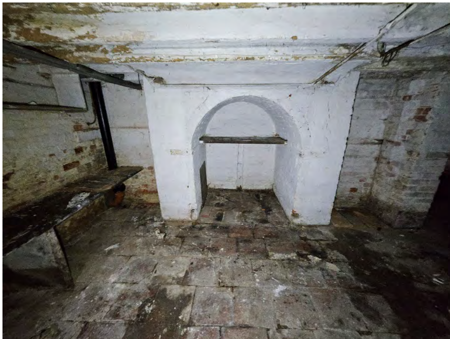
P56 Central base to chimney
