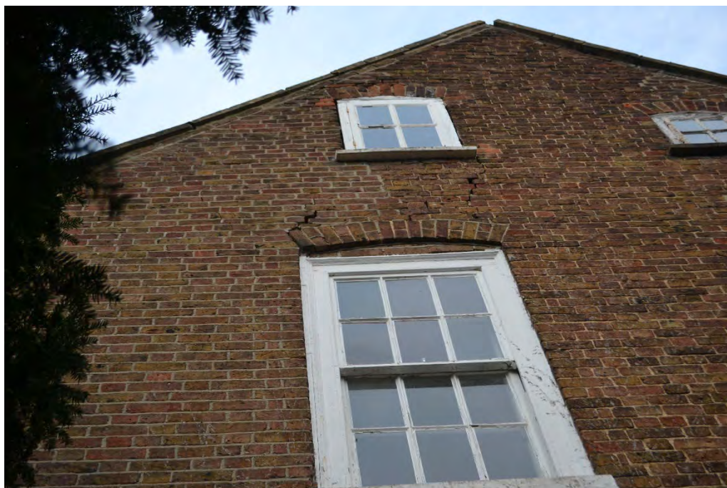
P29 Right-hand elevation – re-pointed brick to front
