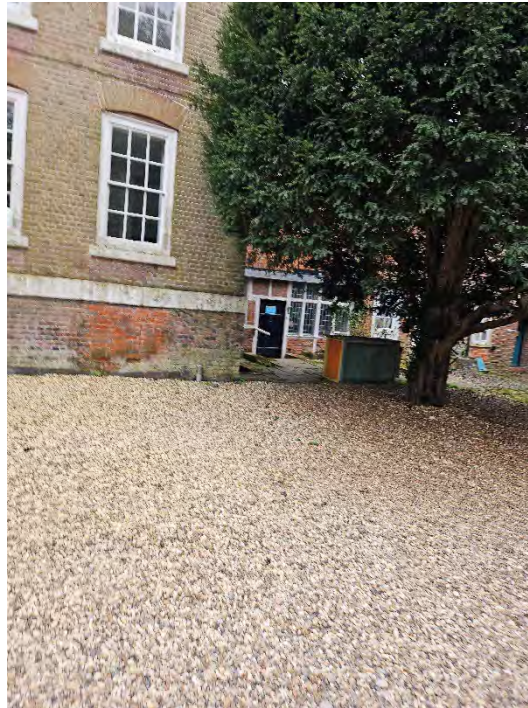
P7 Front right corner – proximity to yew tree
