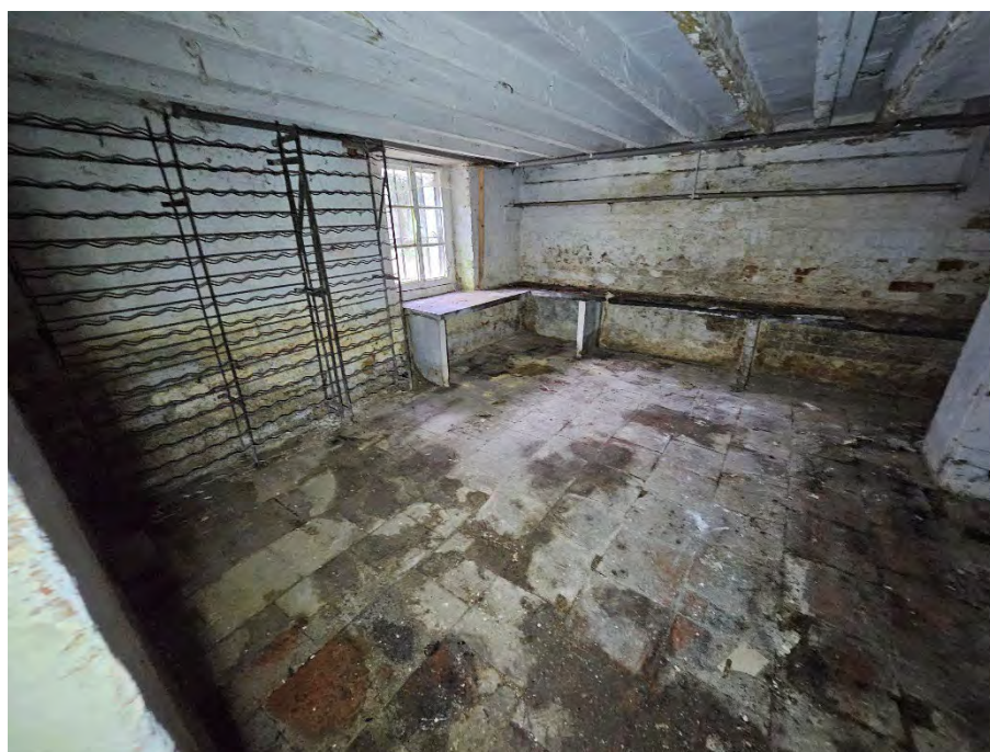
P54 Front left-hand basement room
