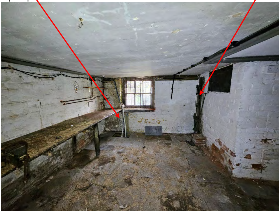
P53 View to rear wall – center of basement
