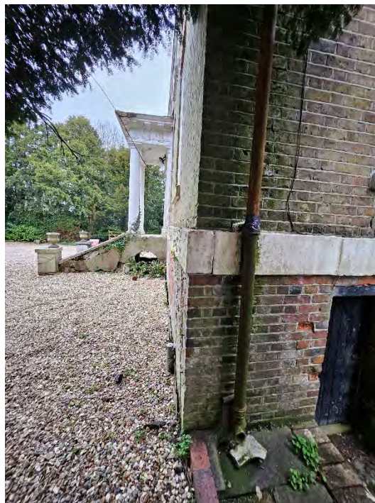
P26 Displacement to corner
