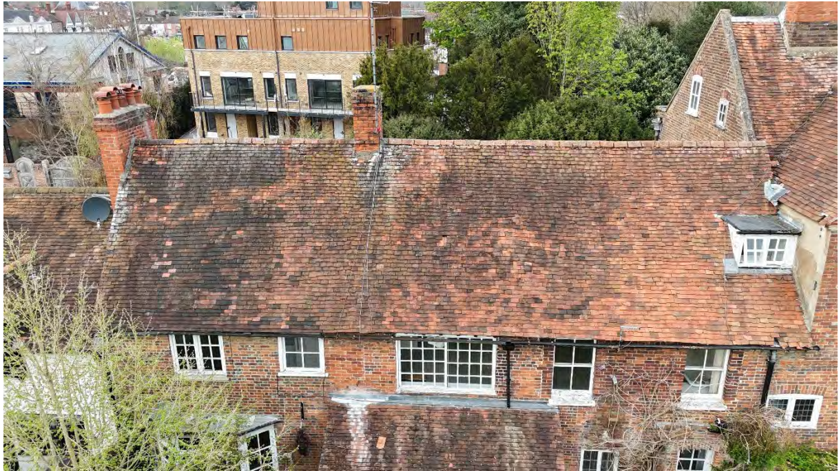
P23 Rose Cottage roof – rear
