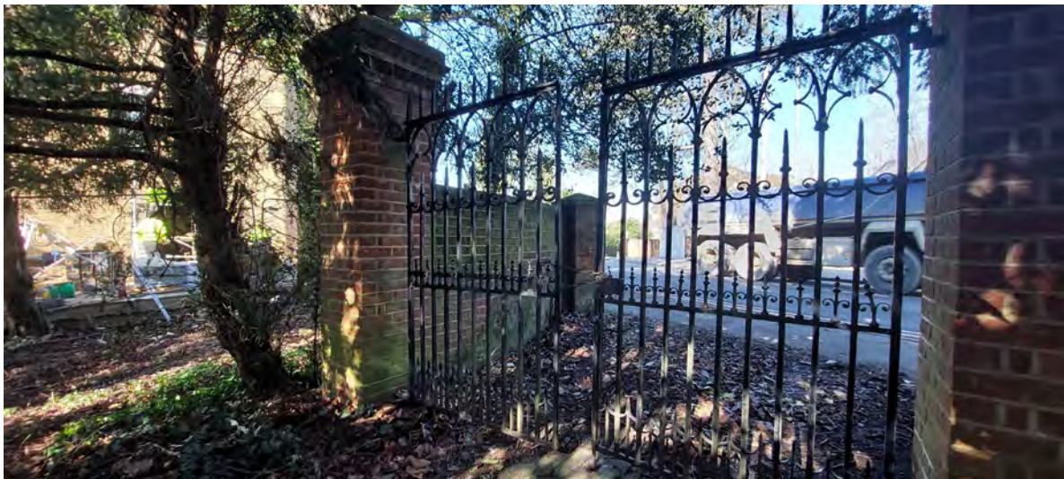
Modern black metal gates, brick wall and gate piers
