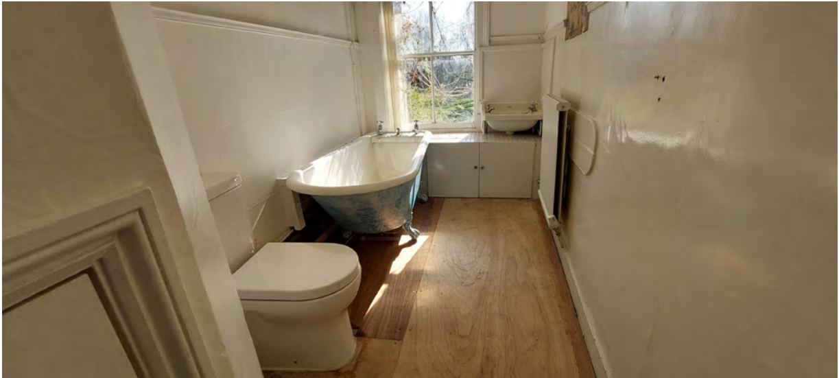
Historic flooring removed
