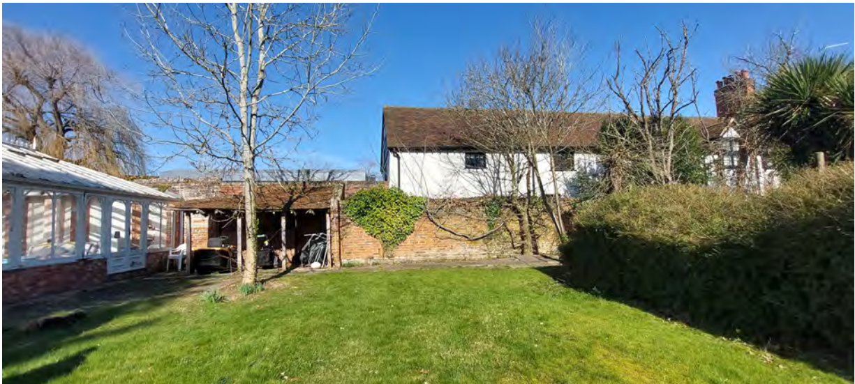
Brick boundary wall along rear of Bird Place Cottage
