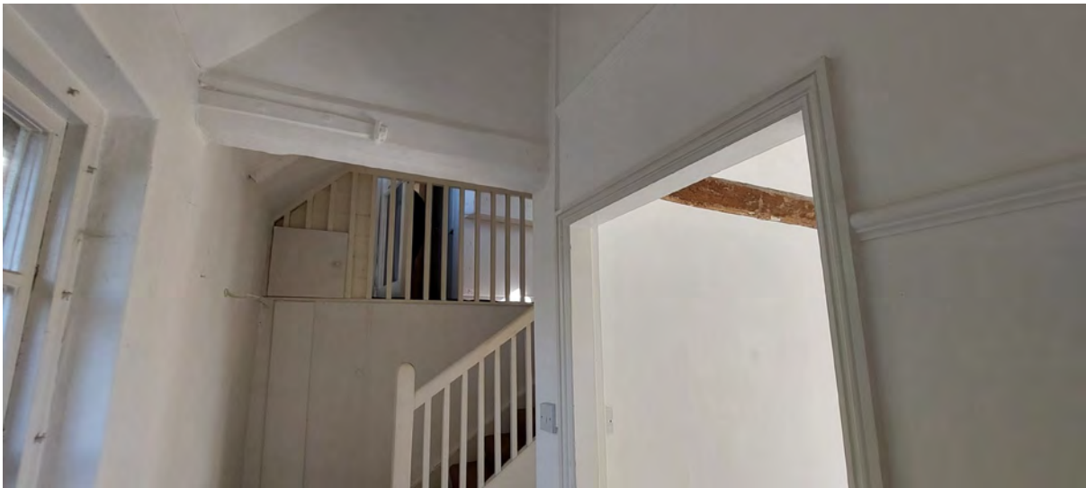
Beams on first floor of Rose Cottage
