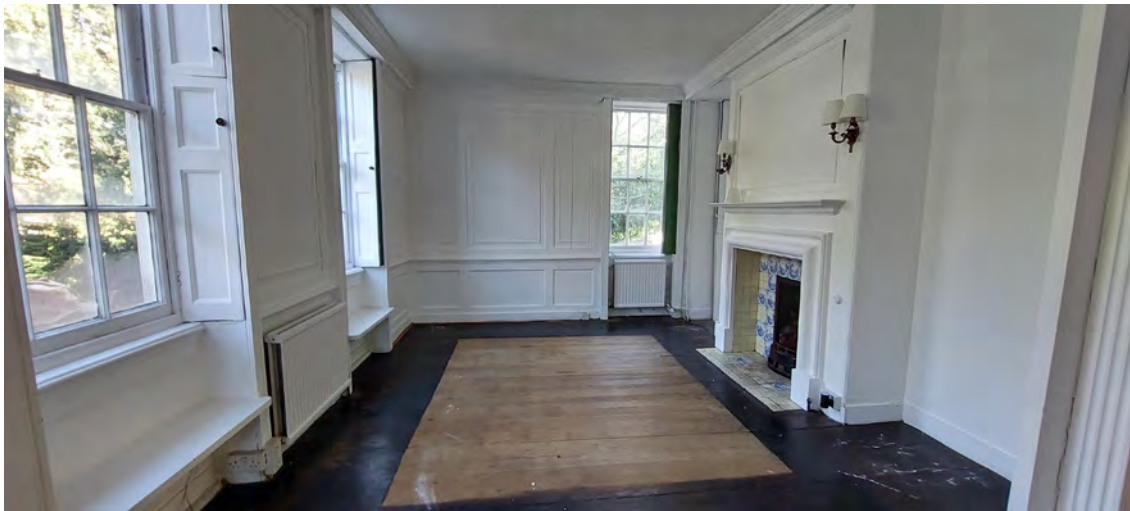
Room at left-hand side of ground floor entrance hall, with historic joinery
