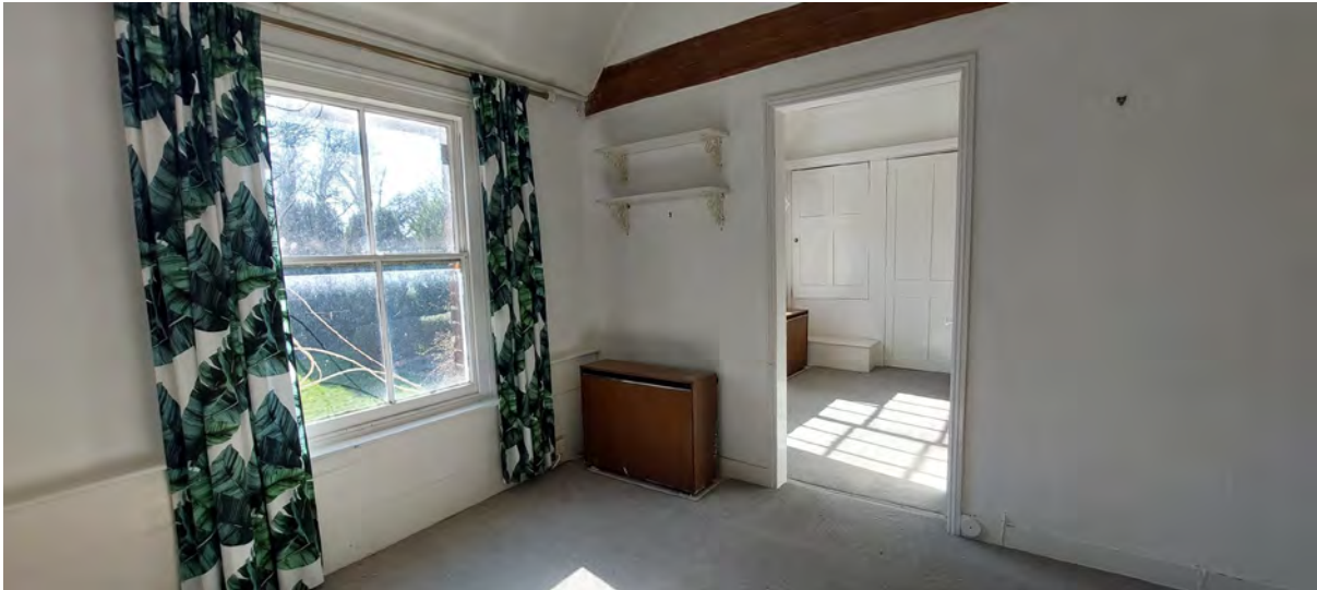
Beams and partition wall on first floor
