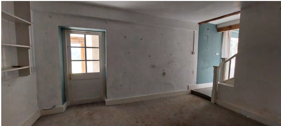
Ground floor of main house where it connects to Rose Cottage
