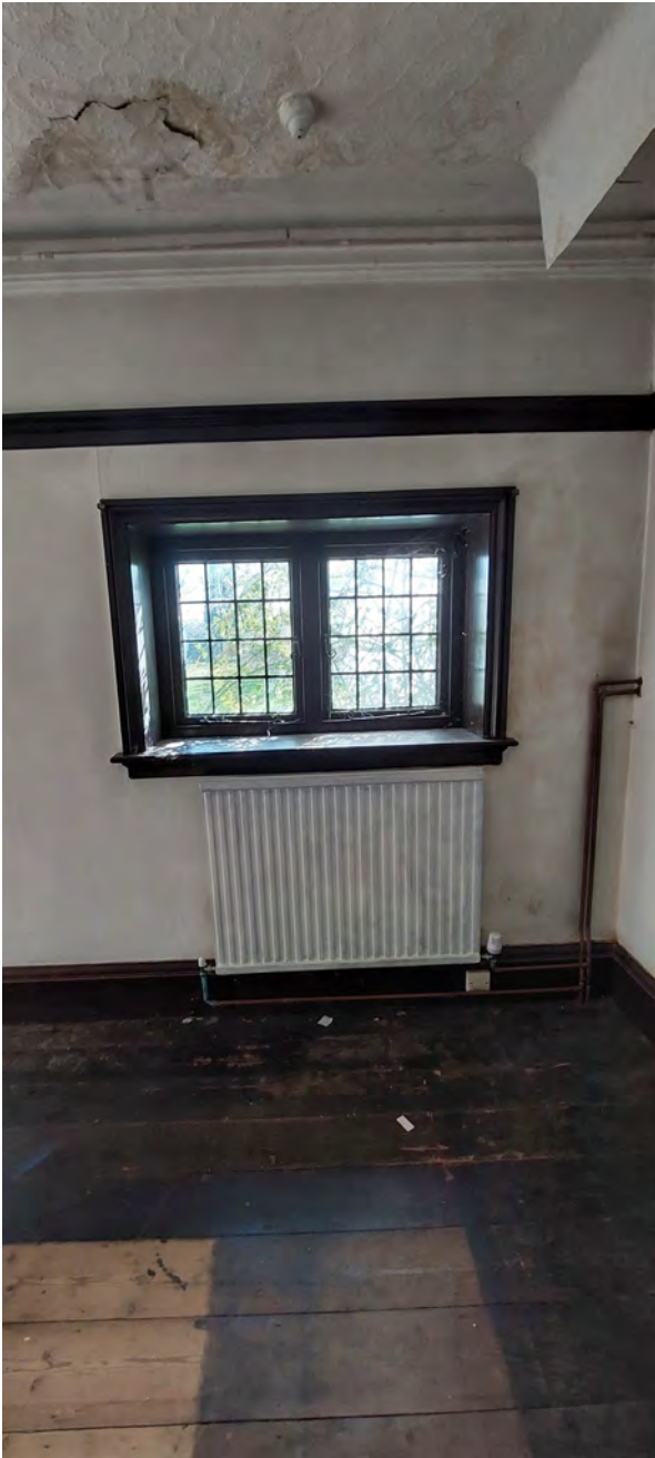
Damaged ceiling and wall plaster in ground floor drawing room
