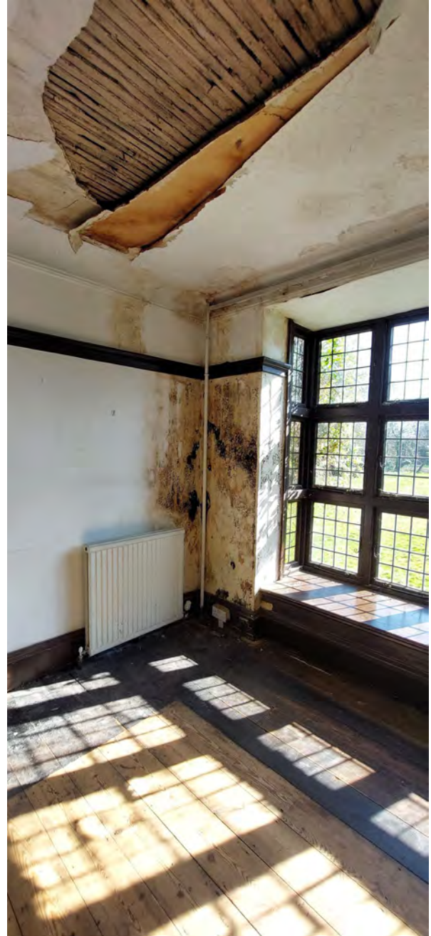
Damaged ceiling and wall plaster in ground floor drawing room
