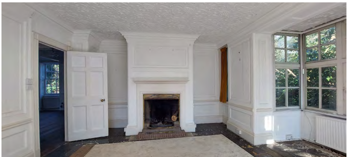
Historic panelling, cornicing, skirting and fireplace in ground floor garden room
