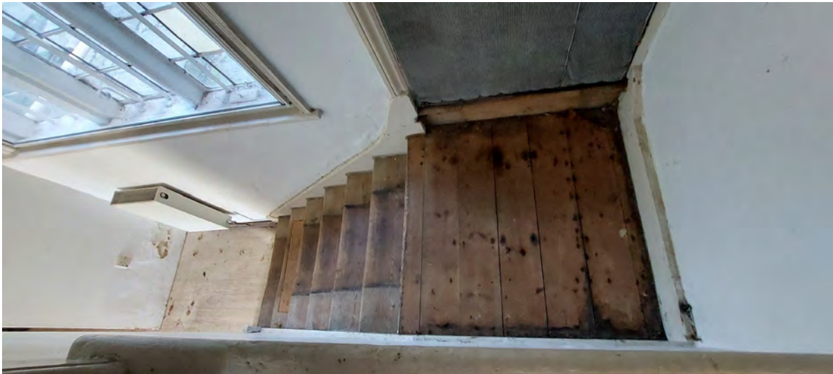
View through service hatch to service stairway leading down to kitchen
