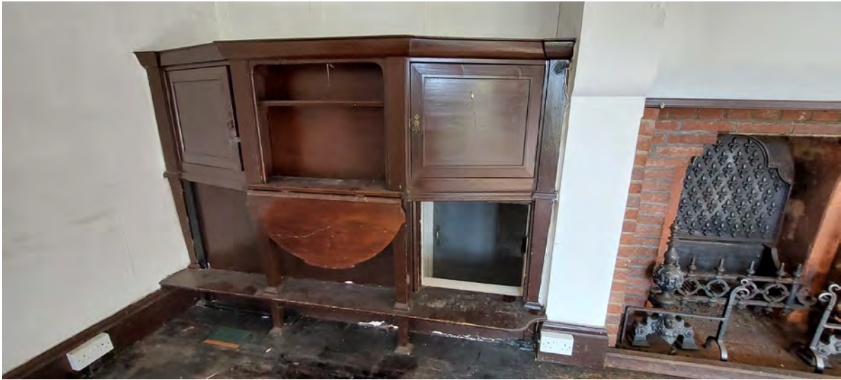
Built-in joinery with service hatch and original fireplace to right
