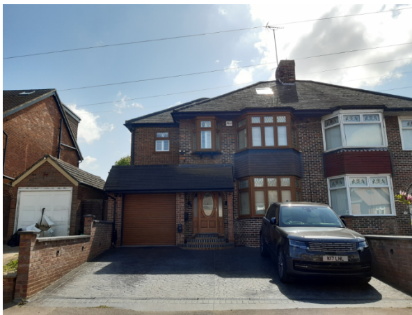
Figure 1 Site visit photo taken 21/04/2026
