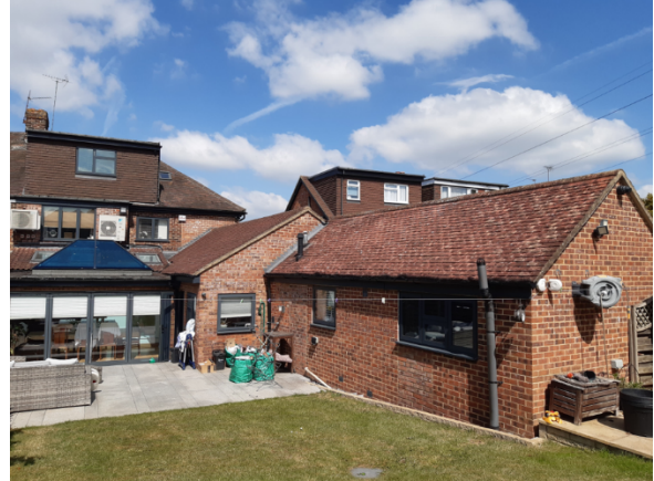
Figure 4 Site visit photo taken 21/04/2026
