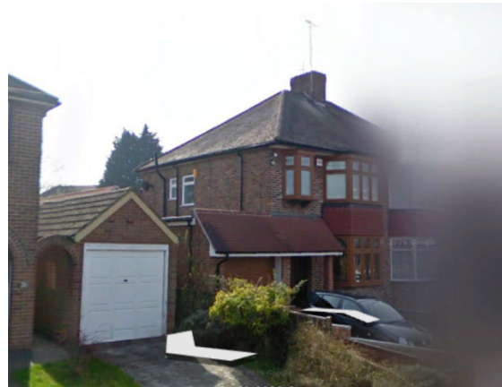
Figure 6 Google Earth Street View 03 2009 showing garage with flat roof and dummy pitch roof to front that differs from approved plans ref 050562.
