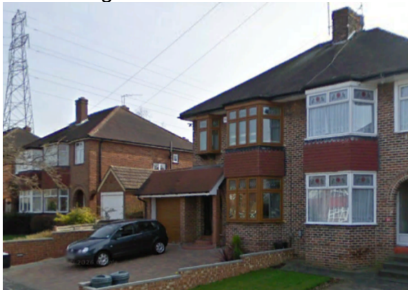
Figure 5 Google Earth Street View 03 2009 showing garage with dummy pitch roof to front that differs from approved plans ref 050562.
