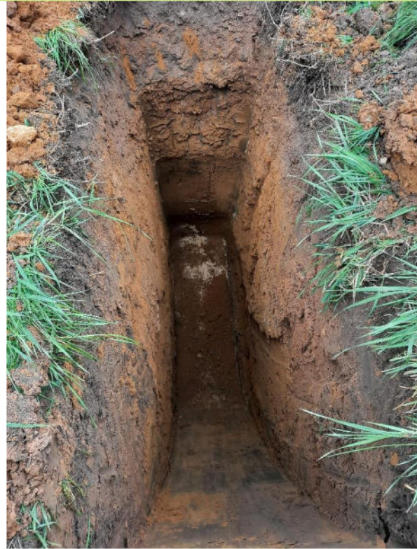
Plate 14 – View of trial pit from above.
