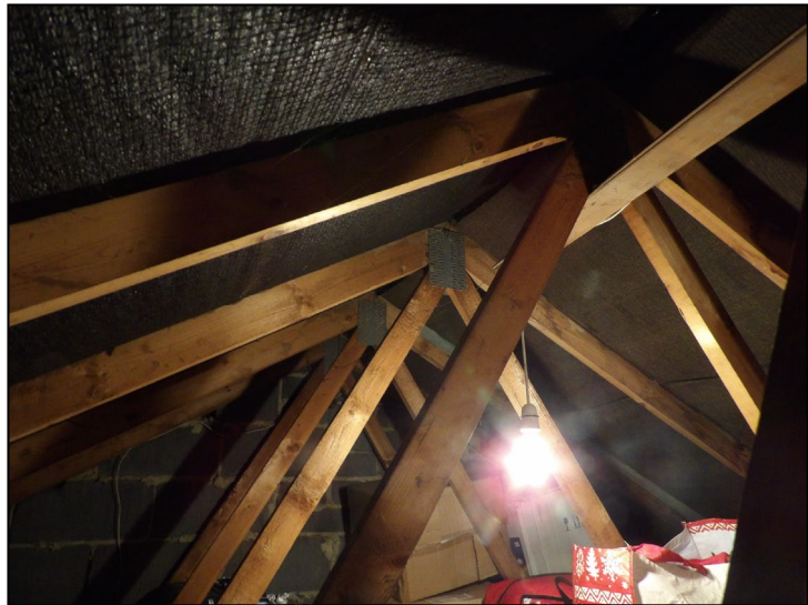
Figure 14. Example bitumen lining to tiles. 23 Starmead Drive, Wokingham. 17.06.25
