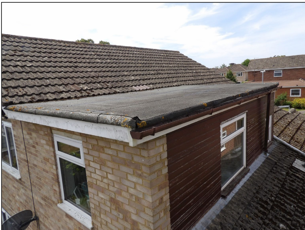
Figure 12. Bitumen covering on dormer roof. 23 Starmead Drive, Wokingham. 17.06.25
