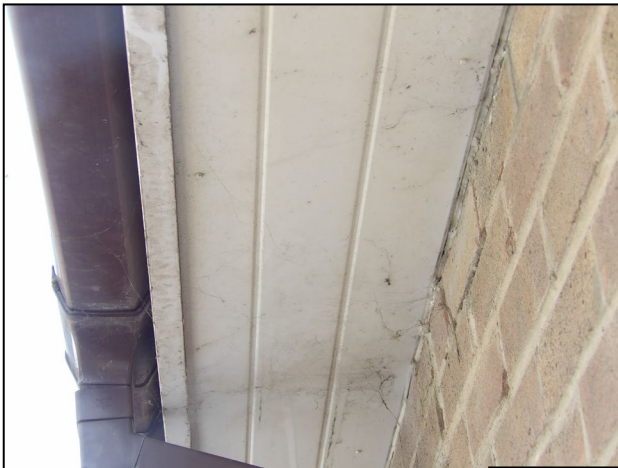
Figure 8. Example sealed soffits/fascias. 23 Starmead Drive, Wokingham. 17.06.25
