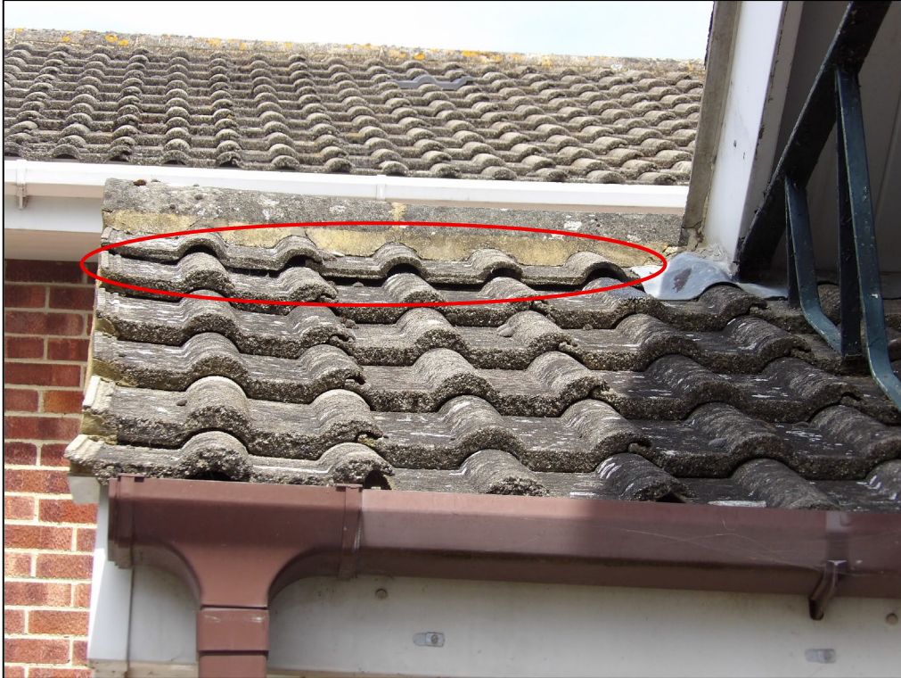
Figure 7. Example gaps in tiles on single storey front pitched roof. 23 Starmead Drive, Wokingham. 17.06.25
