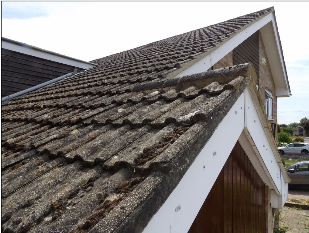
Figure 6. Front view of property and single storey pitched section of roof over part integral garage. 23 Starmead Drive, Wokingham. 17.06.25
