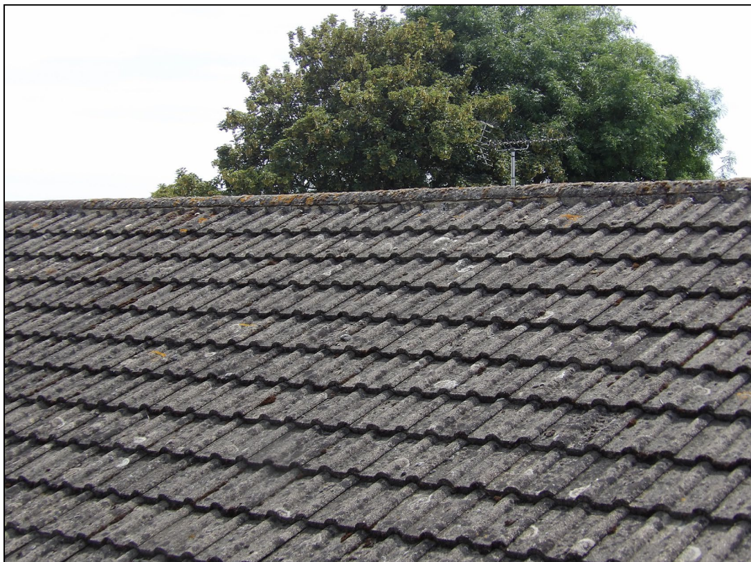
Figure 4. Example of roof and ridge tiles. 23 Starmead Drive, Wokingham. 17.06.25
