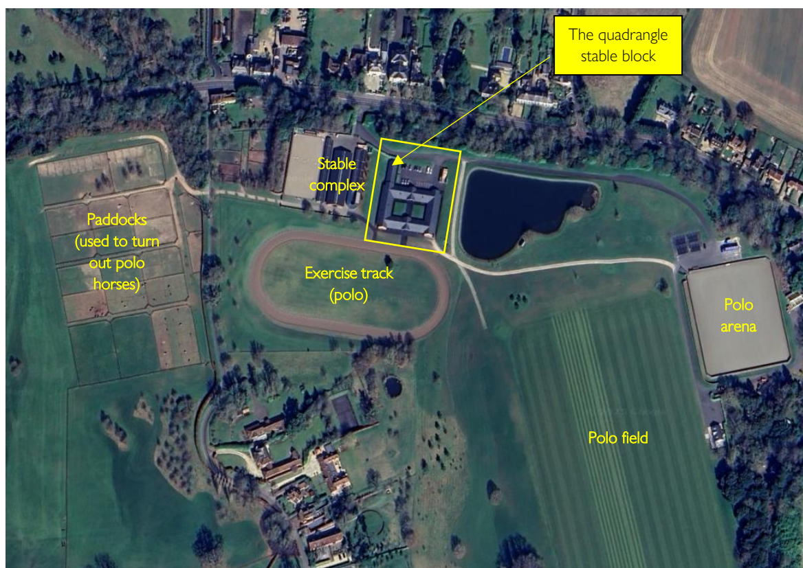
Fig. 1 – Latest aerial view (dated 2025) showing the location of the polo facilities, stables and paddocks
