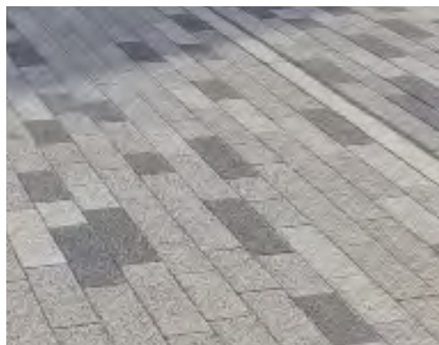
Textured paving with conservation kerb
