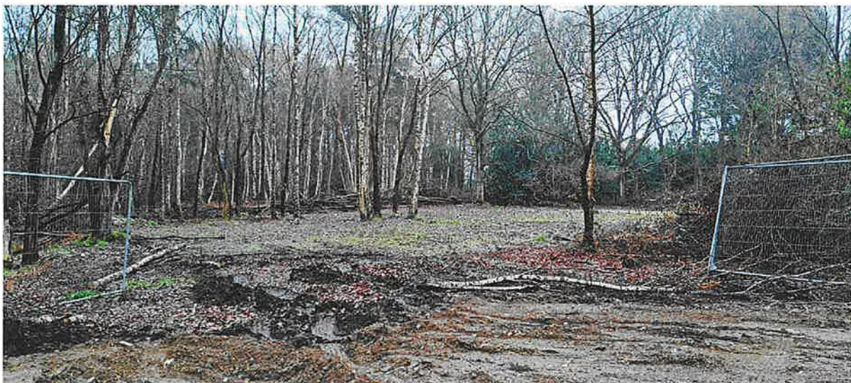
Picture 3 After clearance of site
