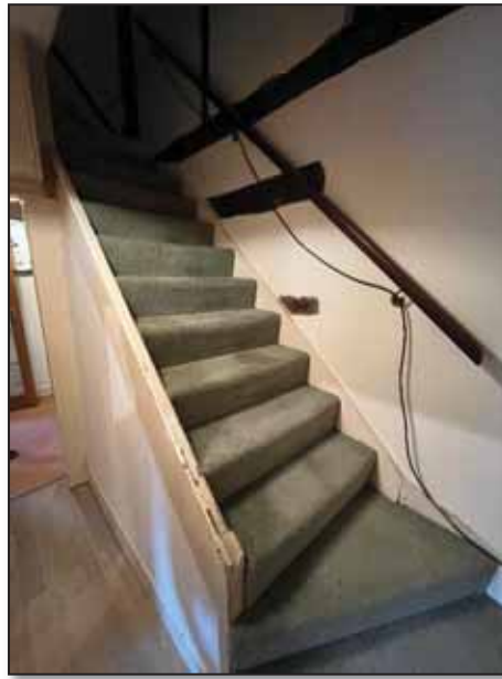
Image 15: Existing stairs to first floor
