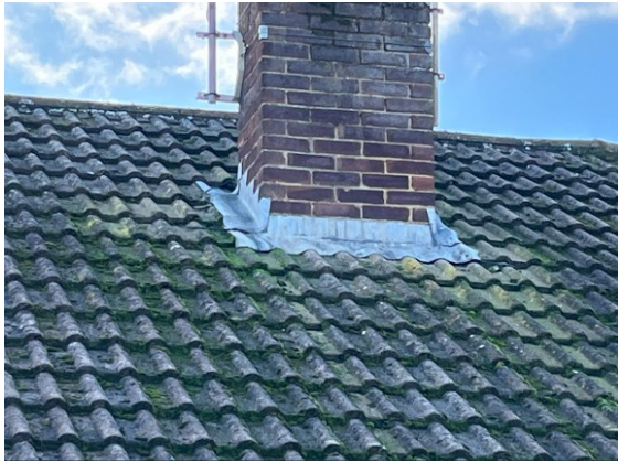
Photograph 10. Lead flashing sealed to chimney and roof tiles (rear elevation).
