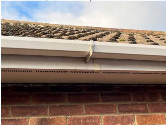
Photograph 12. Vented uPVC soffit sealed to the brickwork (southeast elevations).
