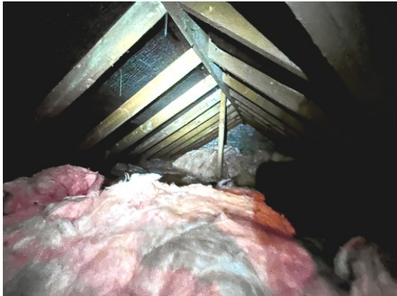
Photograph 14. Fully intact bitumen felt roof lining.
