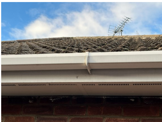
Photograph 7. Fully intact hip mortar (southeastern elevation).
