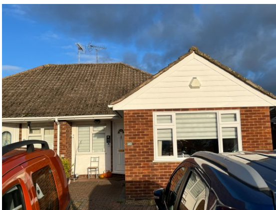
Photograph 1. Front elevation viewed from the southwest.
