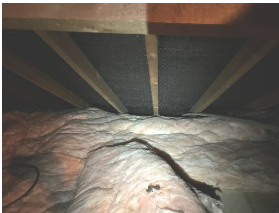
Photograph 16. Open eaves with access to the vented uPVC soffit.
