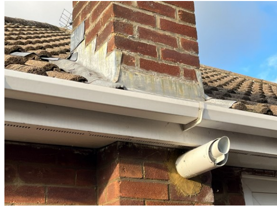
Photograph 11. Lead flashing sealed to chimney and roof tiles (southeast elevation).
