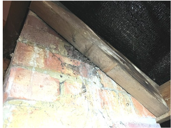
Photograph 15. Timbers sealed to the brickwork chimney.
