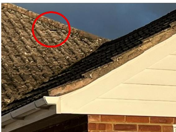
Photograph 3. Sealed interlocking roof tiles (rear elevation).
