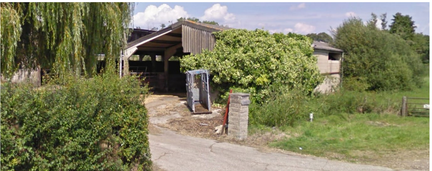
Figure 3: Google Street View imagery, August 2011
