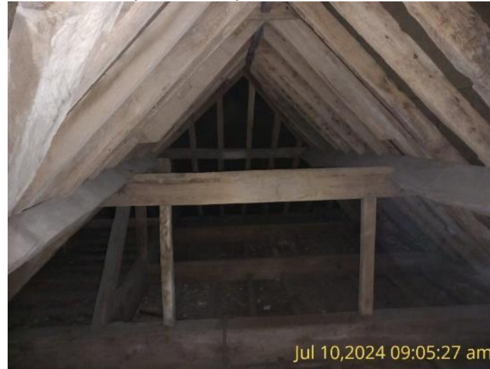
Figure 2: L1 – Loft space within the interior of B1.
