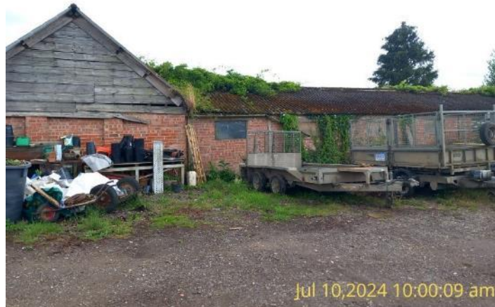
Figure 4: B4 – Northwest elevation.
