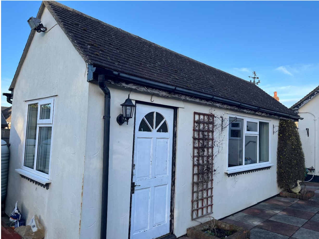
Figure 10. Garage looking north
