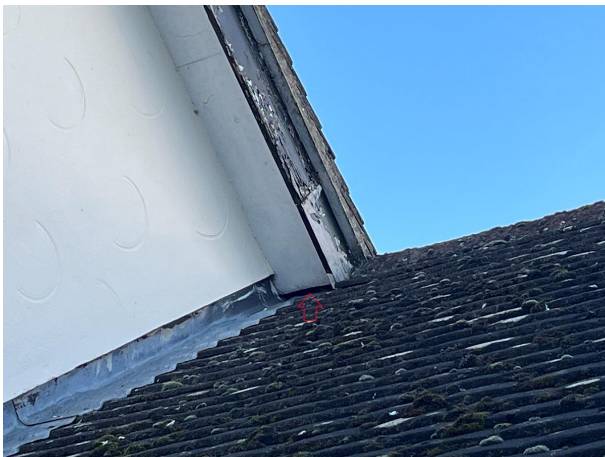
Figure 4. Detail of opening into soffit on rear of property: Red arrow indicates potential openings for roosting bats.
