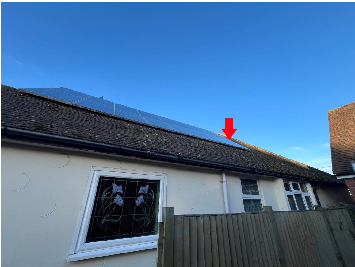
Figure 6. South face of roof looking east: red arrow indicates potential openings into undertile spaces (see figure 7)
