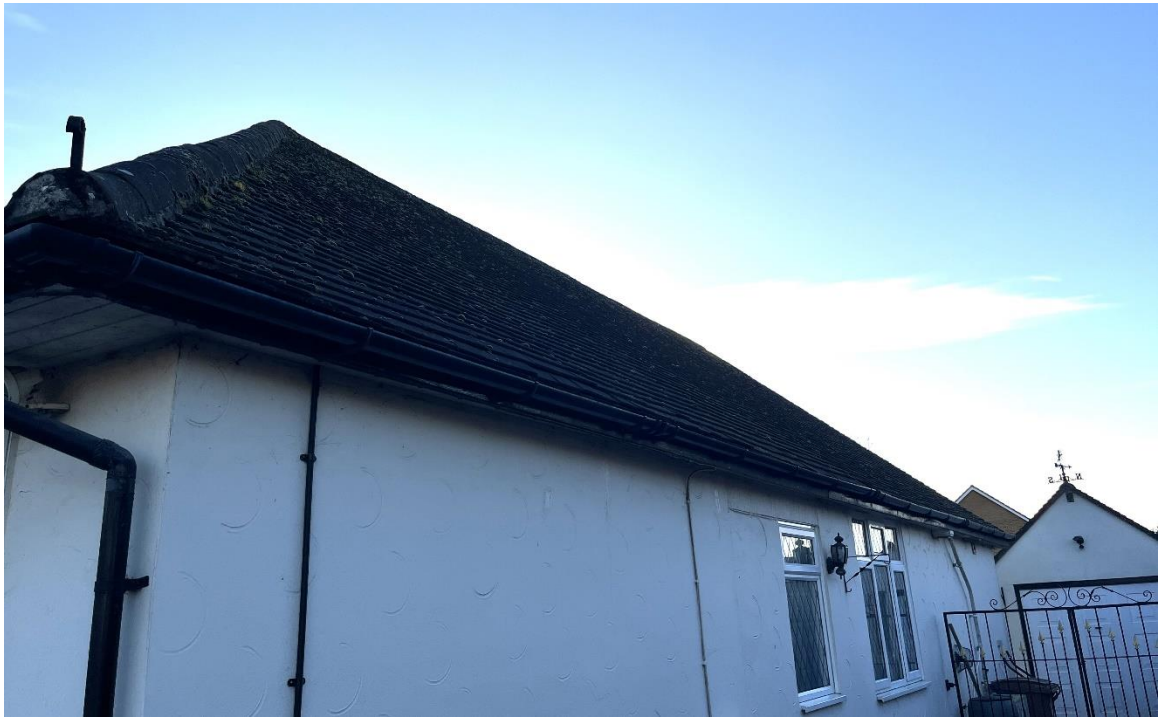
Figure 5. Northern elevations looking west.
