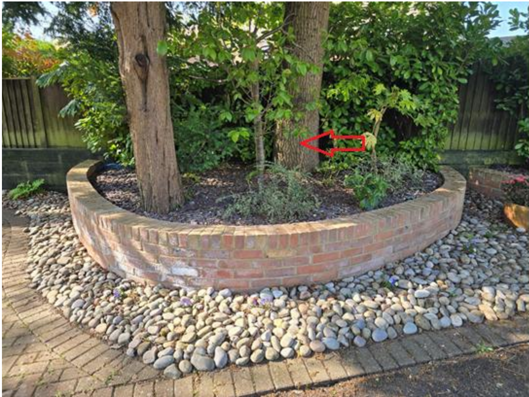
Photo 1 – Raised brick retaining wall at base
