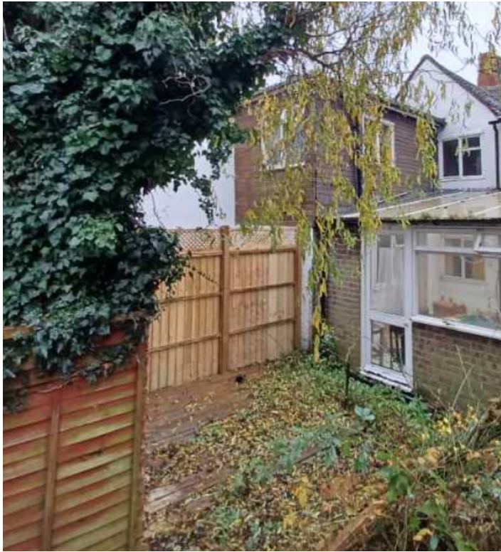
Vertical close boarded fence off kitchen to No.38 does appear to belong to belong to 3 Rose Court.
