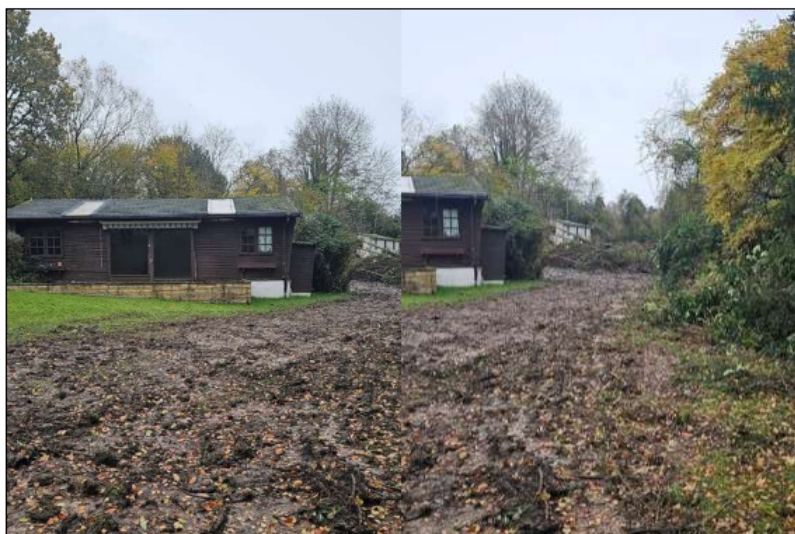
TN 1: Timber clad shed.
