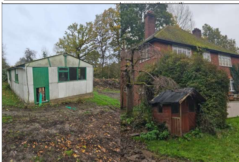
TN 15: Wooden outbuilding.
