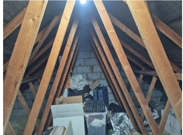
Photograph 7: Loft of B1.
