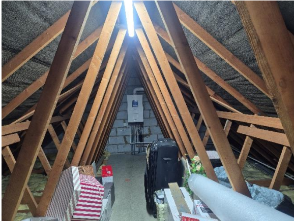
Photograph 6: Loft of B1.
