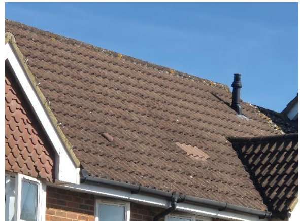
Photograph 9: Roof on the southern elevation of B1.
