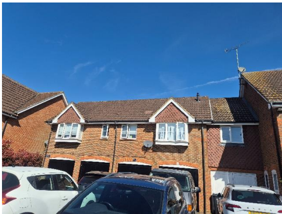
Photograph 1: Southern elevation of B1.
