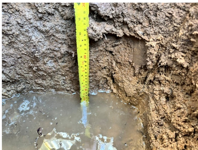
Photo 1 – Excavation with Ground Water
