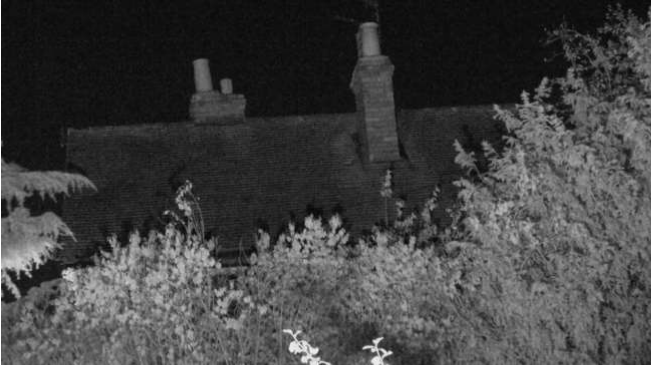
Photograph 3 – southern elevation of the property.
