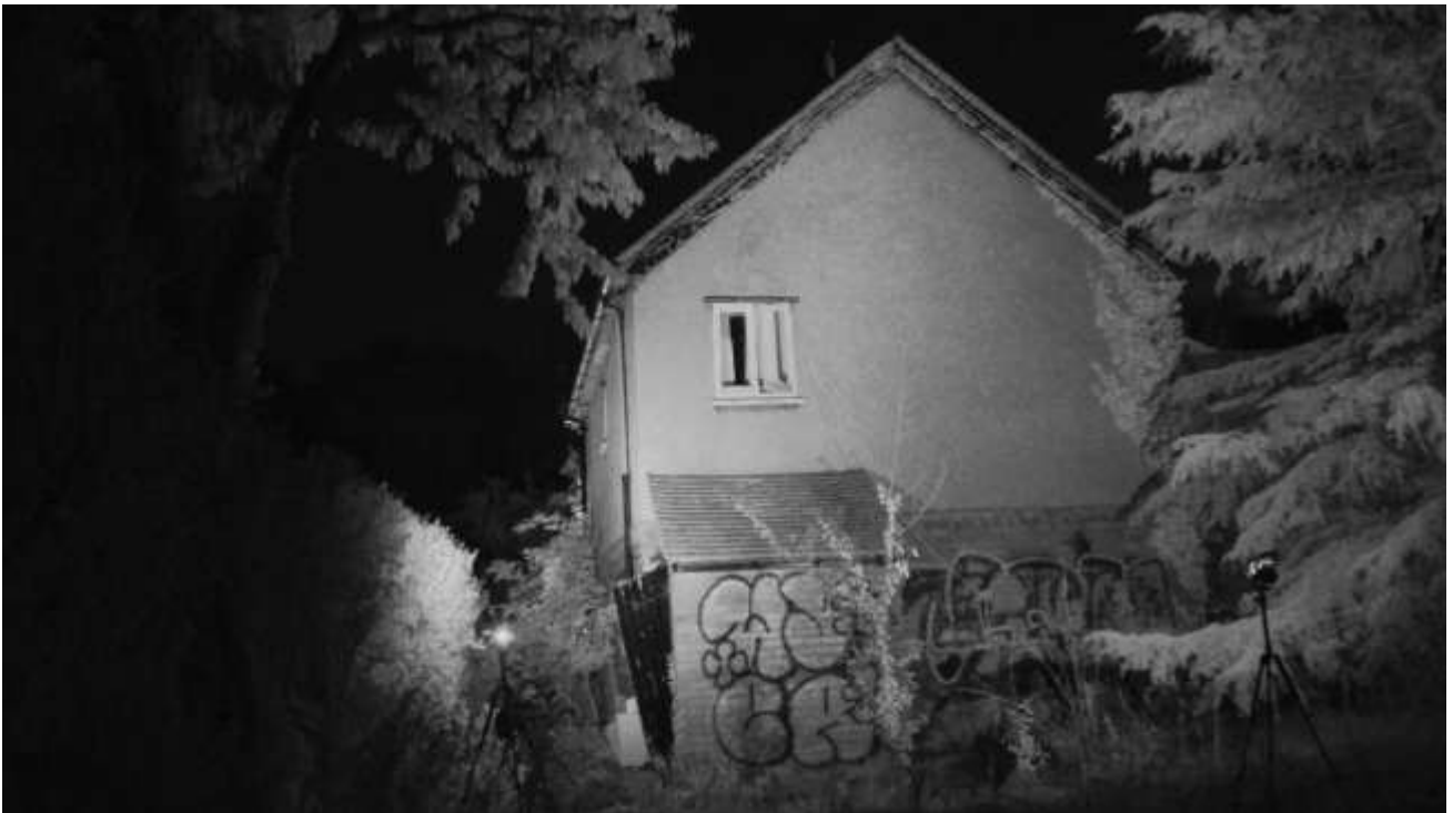
Photograph 2 – western elevation of the property.
