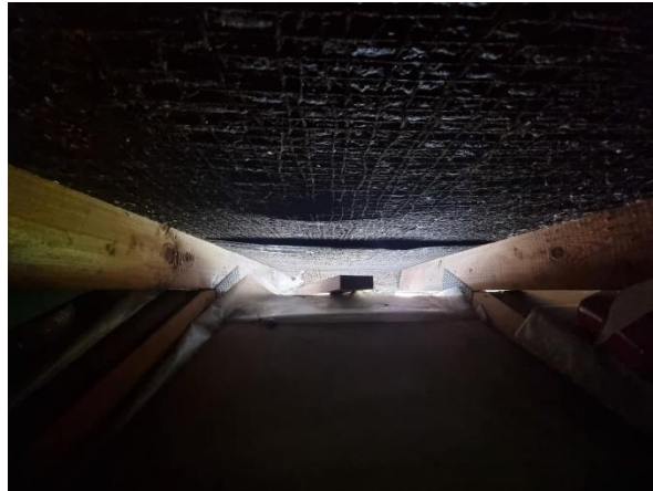
Figure 5. A gap between the soffit and sarking felt.
