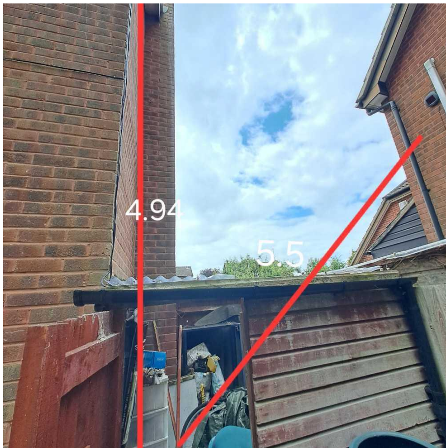
Rear elevation - showing existing structure in relation to Number 2 Adams Way
