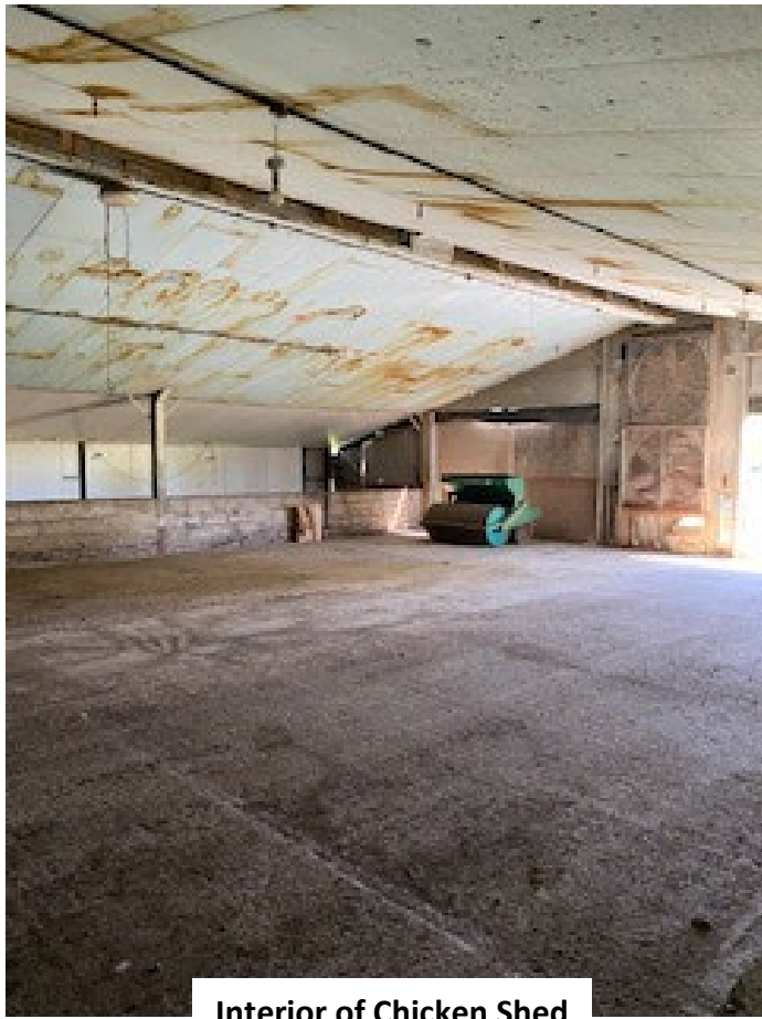
Interior of Chicken Shed
