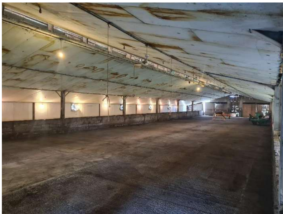
Photograph 14: Internal view of the former chicken shed
