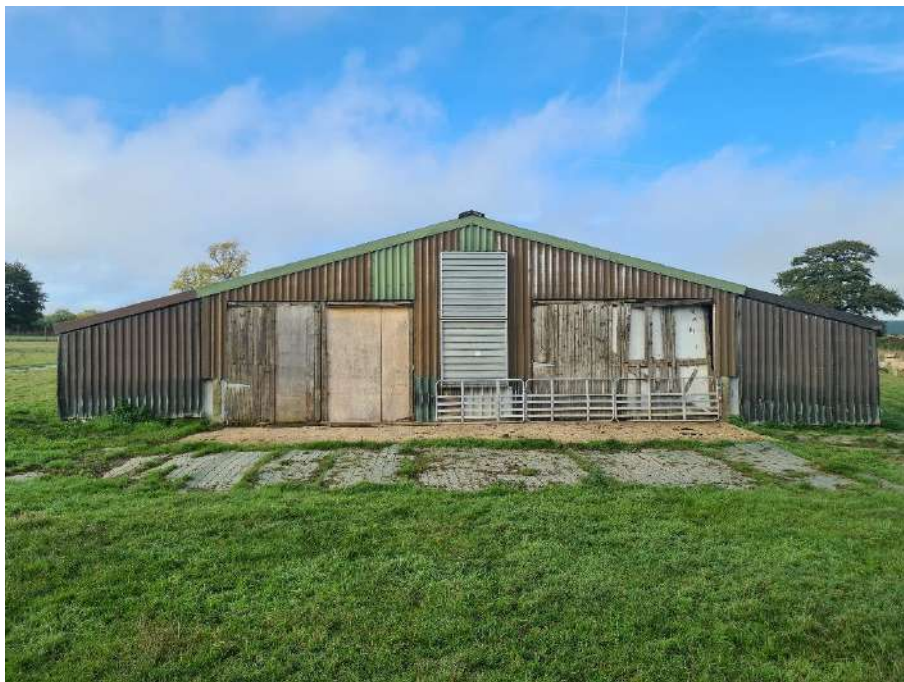
Photograph 8: A view showing the northern elevation of the barn.
