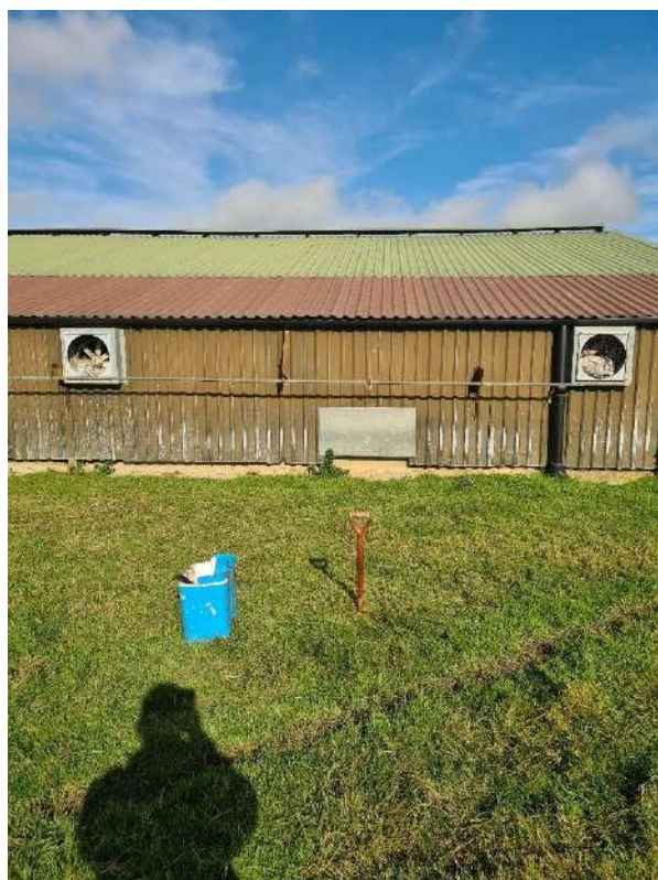
Photograph 21: Sampling along the eastern elevation of the building.
