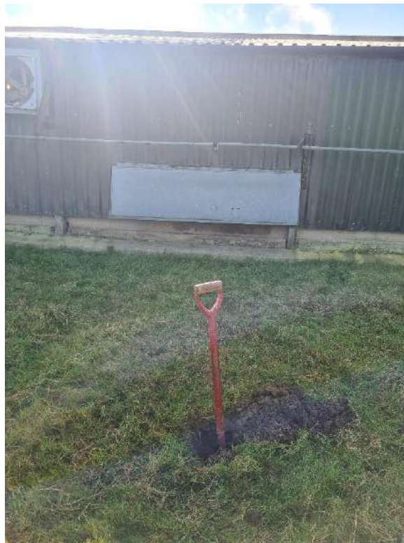
Photograph 19: Hand digging to obtain a sample for testing outside one of the chicken doorways.
