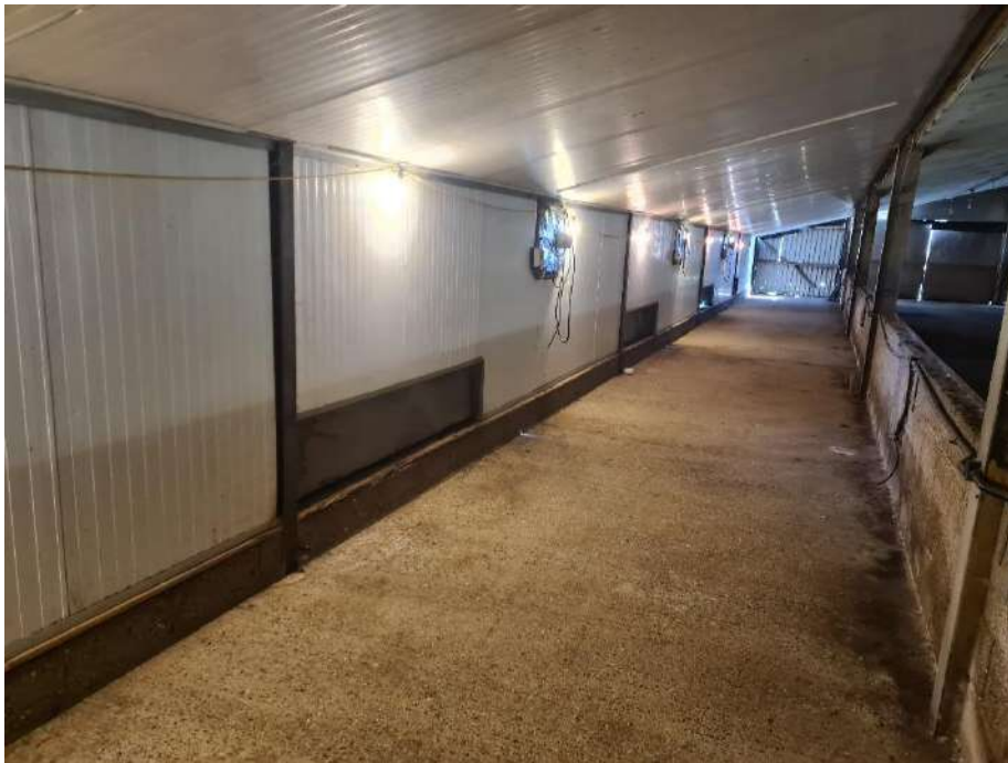
Photograph 17: Extended side section to the barn. Note extension of concrete slab across entire area.
