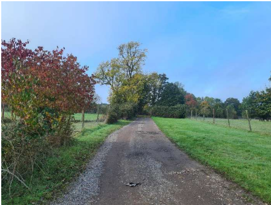
Photograph 1: A view of the access track leading from Binfield Road towards the barn.
