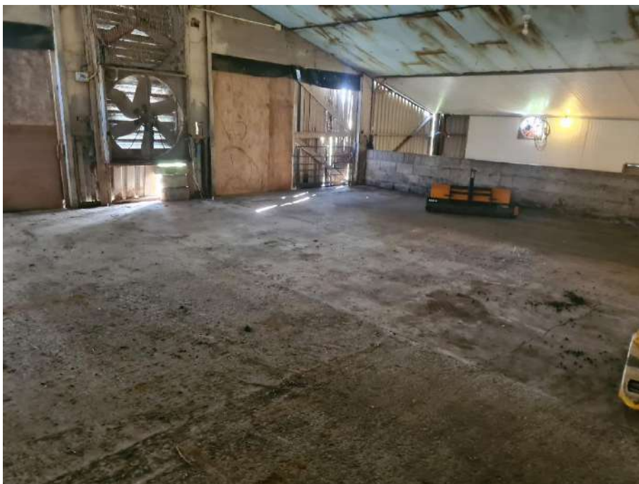
Photograph 18: Internal area of the northern section of the barn.
