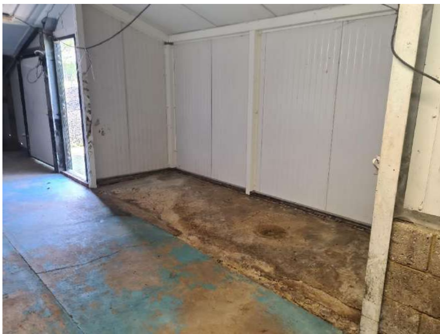
Photograph 12: Internal concrete surfacing near the barn entrance.
