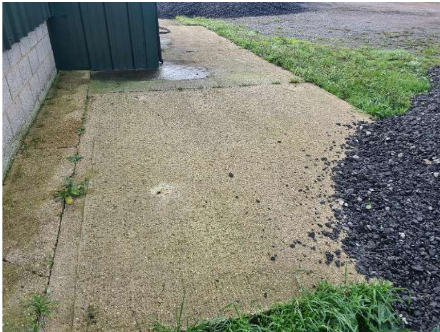
Photograph 5: A view of concrete hardstanding to the front of the barn
