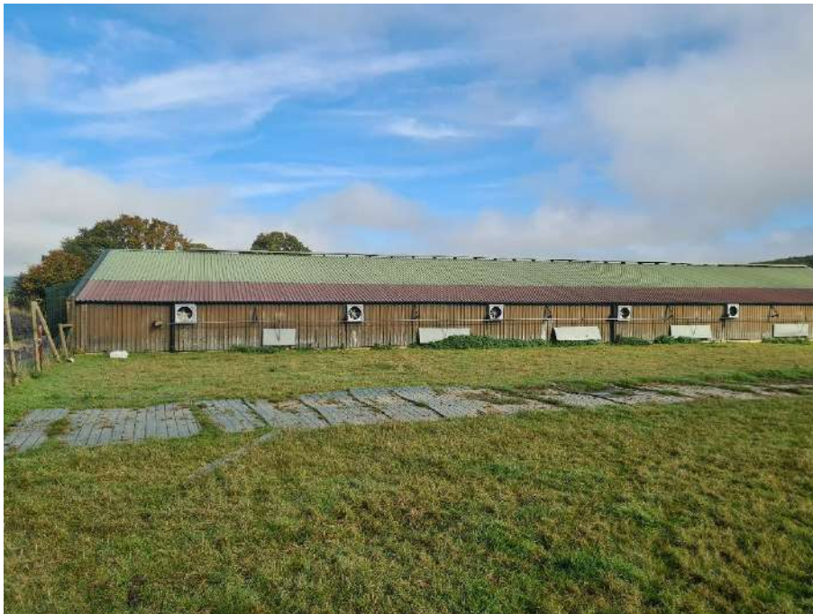
Photograph 11: A further view showing the eastern elevation of the building.
