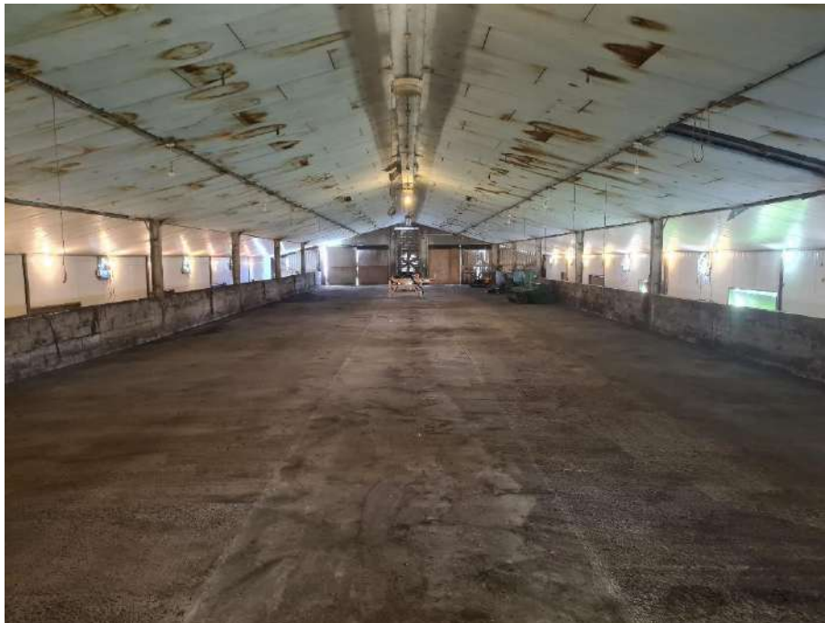
Photograph 15: Further internal view across the barn. Note good quality concrete located throughout.
