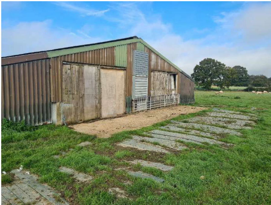
Photograph 9: A view showing concrete strip and plastic matting located outside of the main doorways.
