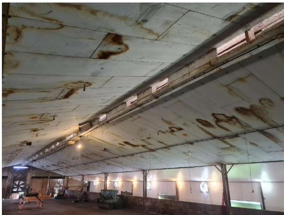
Photograph 16: Internal roofing detail
