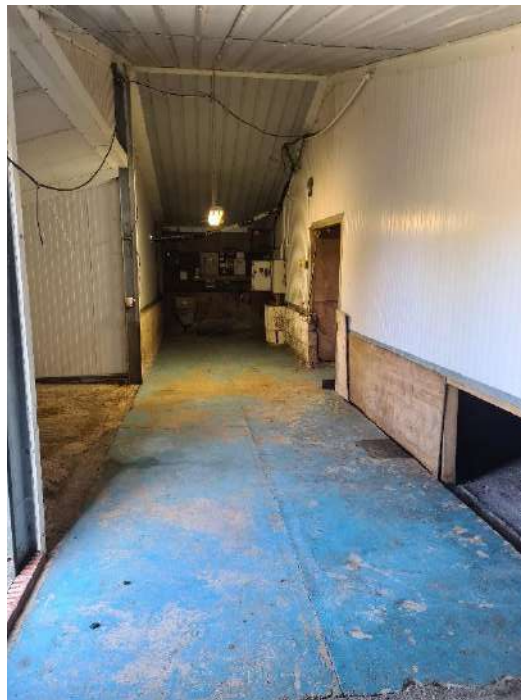
Photograph 13: Painted concrete surfacing noted across the front of the barn.
