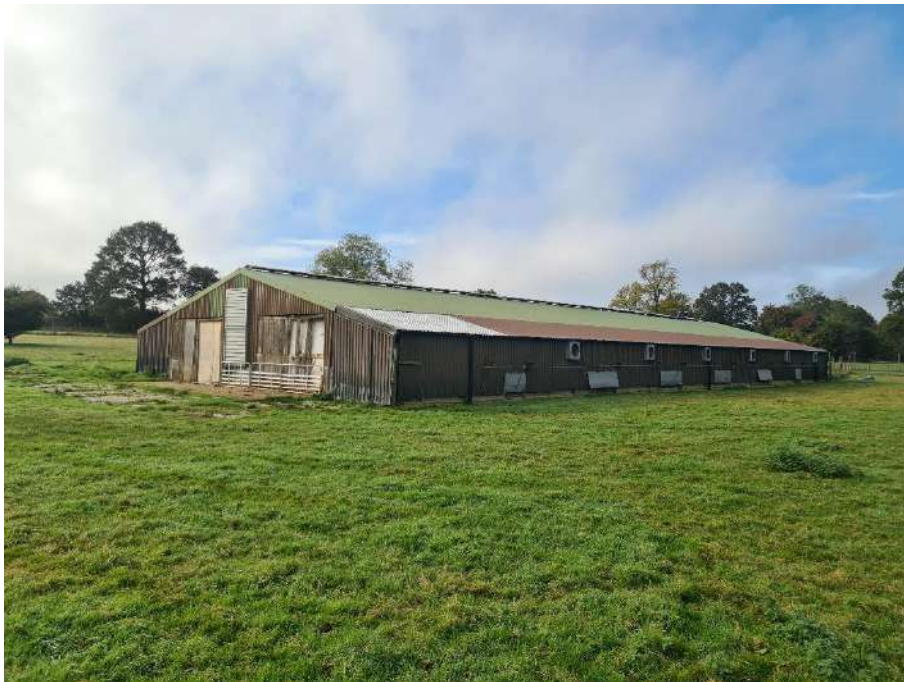
Photograph 7: A view showing the barn as taken from north to south.
