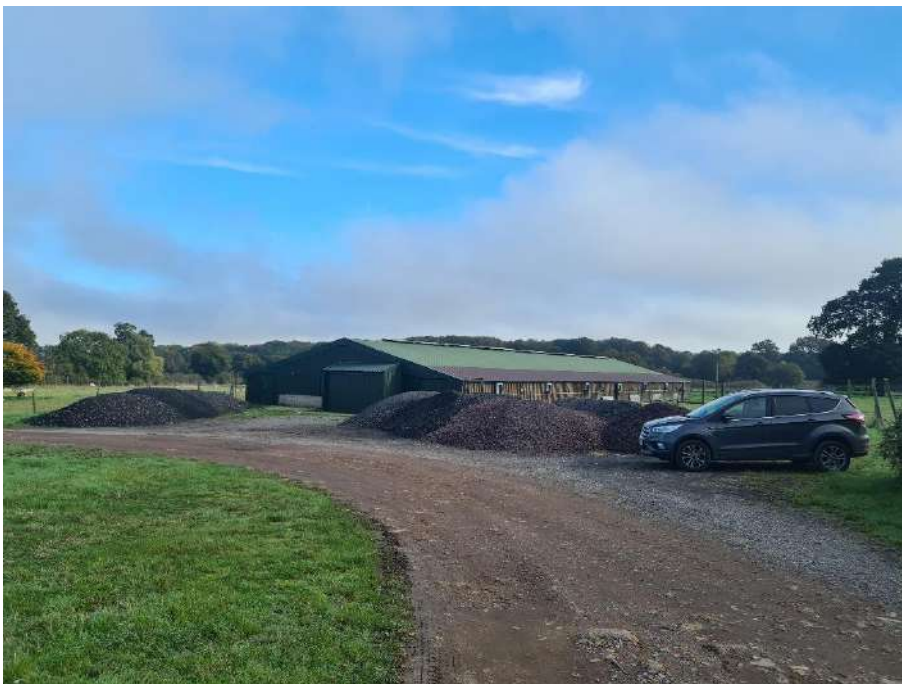
Photograph 2: A view of the former chicken shed
