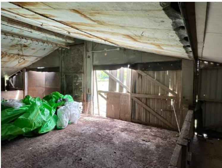
Open rear to Barn
