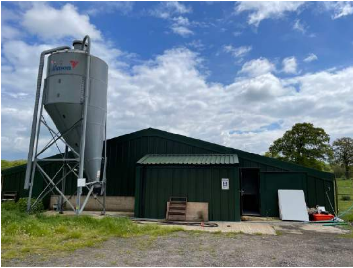
Frontage to Barn
