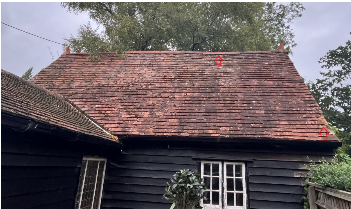
Figure 7. North outbuilding looking north. Red arrows indicate potential openings for crevice roosting bats.
