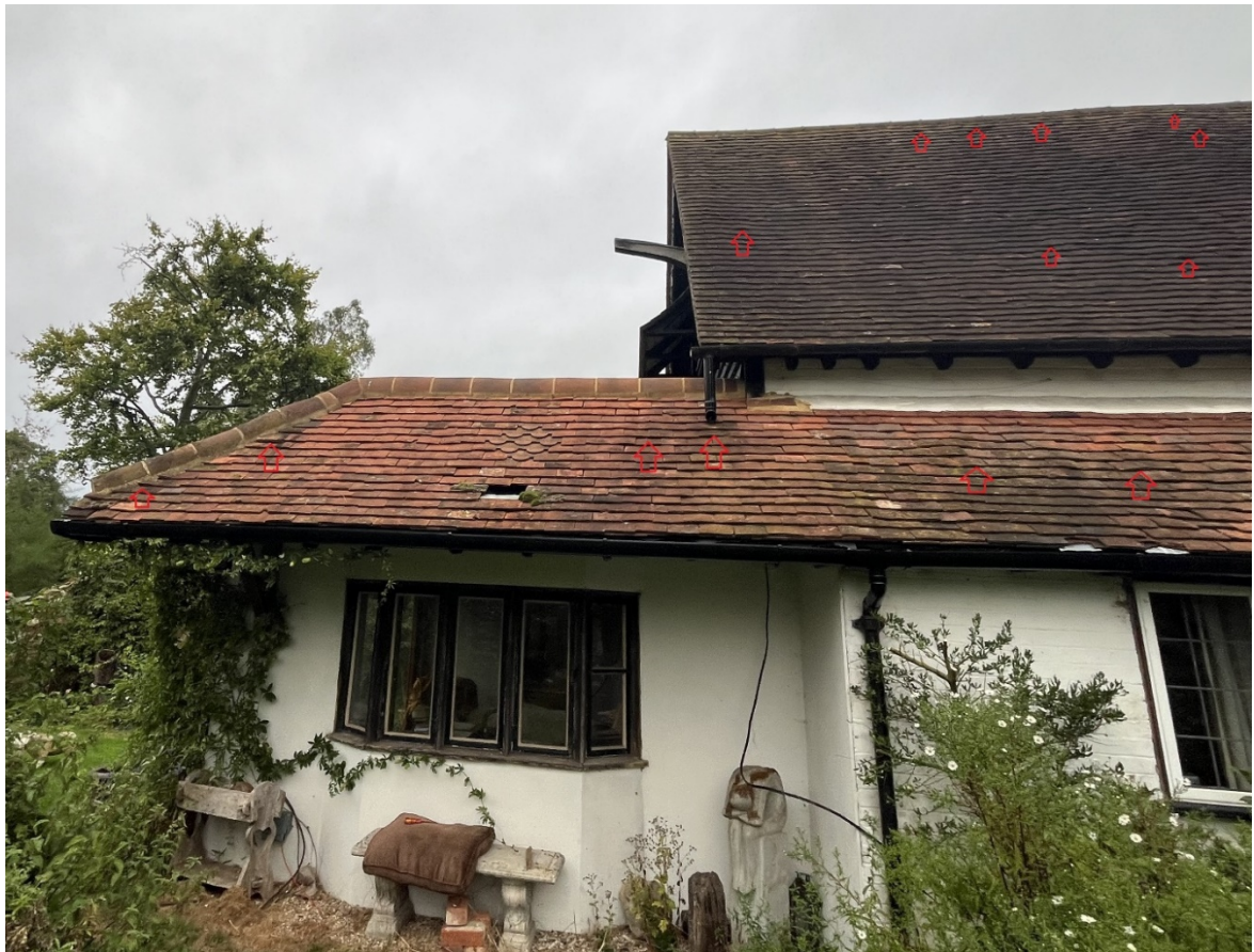
Figure 4. Southern elevations (western half) looking north. Red arrows indicate potential openings for crevice roosting bats.
