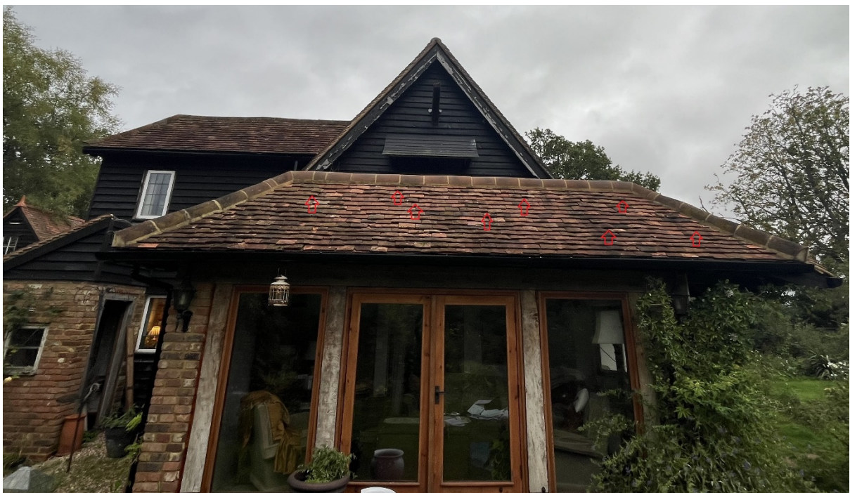
Figure 5. Western elevations looking east. Red arrows indicate potential openings for crevice roosting bats.
