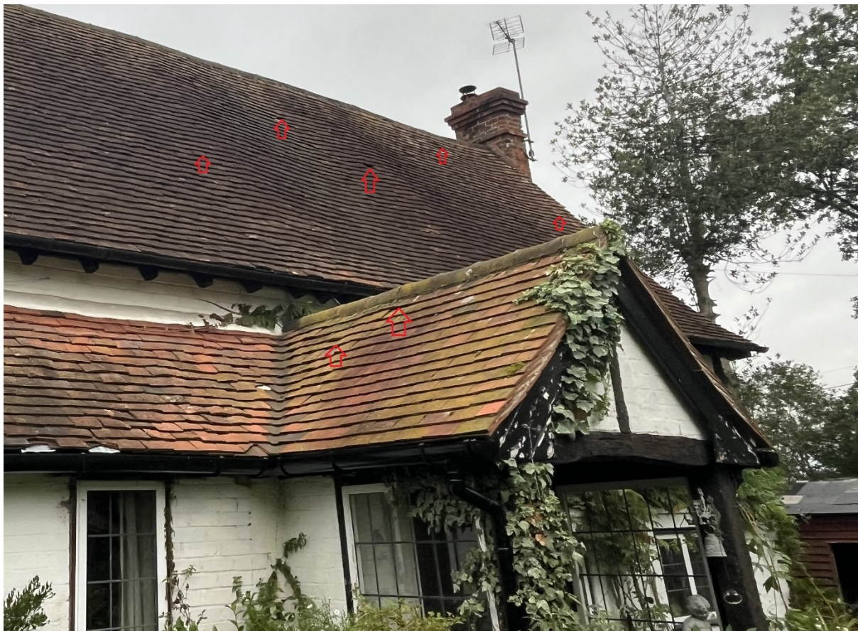
Figure 3. Southern elevations (eastern half) looking northeast. Red arrows indicate potential openings for crevice roosting bats.
