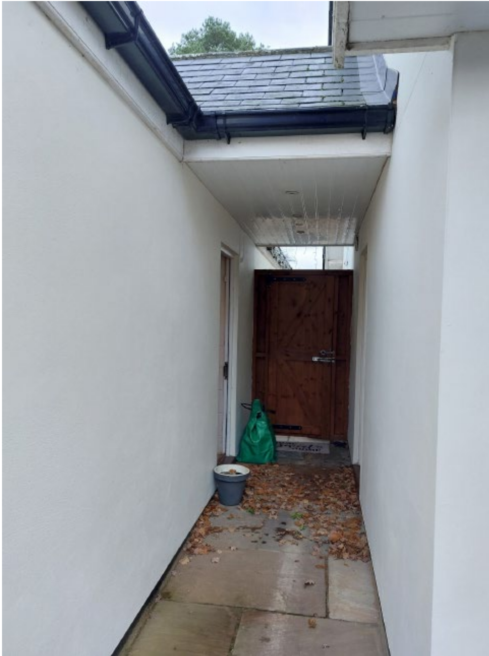
Existing access gate between dwelling and link-attached extension
