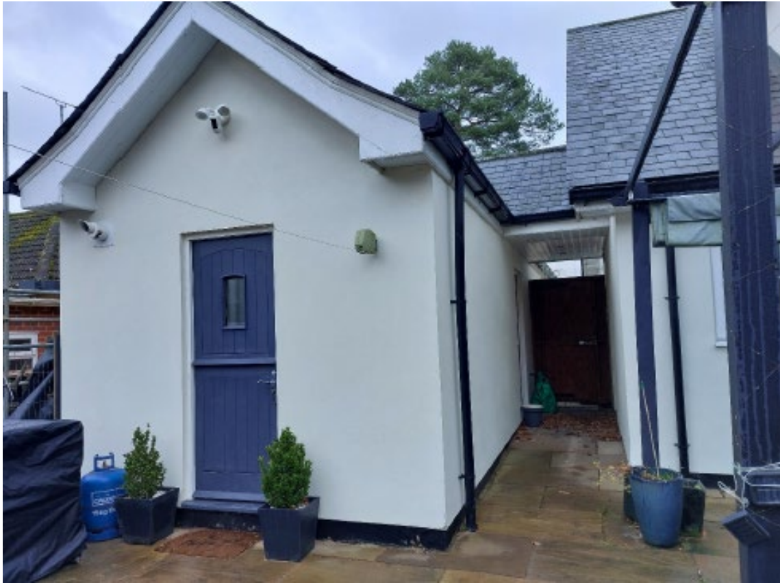
Existing link-attached garage (rear elevation)
