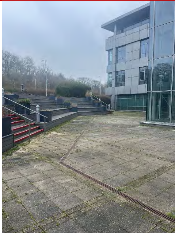
Photo 3 – rear of building 3
