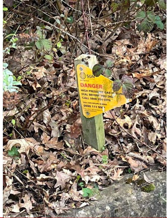
Photo 18 – gas pipeline on southern boundary
