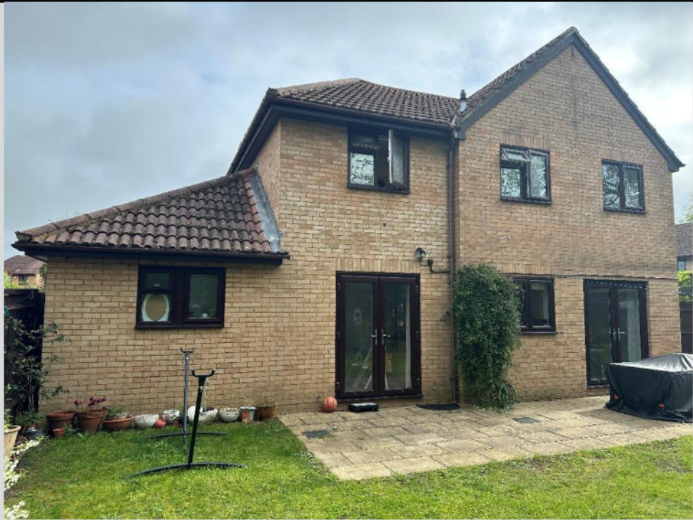
Area where the bedroom extension is to be located
