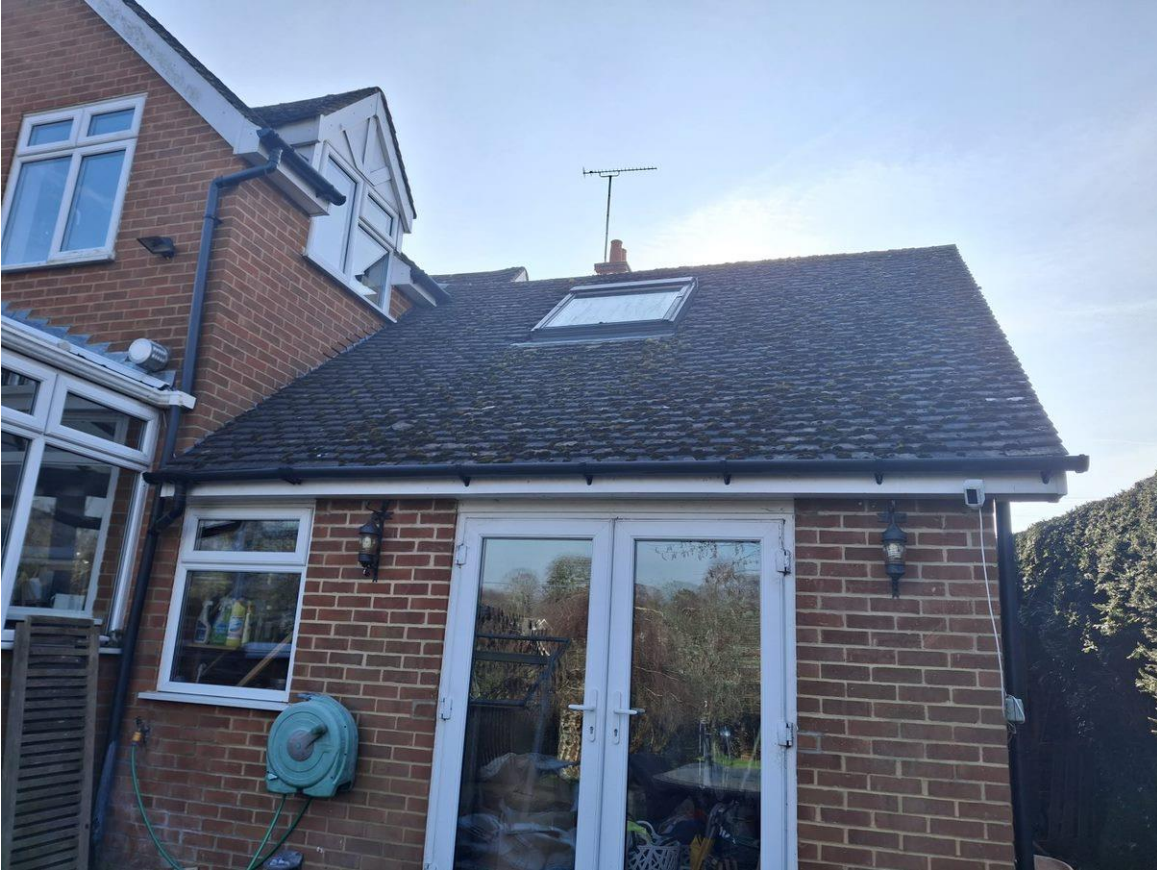
The rear (north) of B1c
