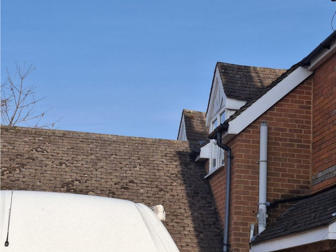
The east roof of B1c meets the west of B1b
