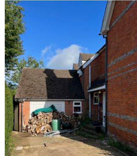
South elevation of garage
