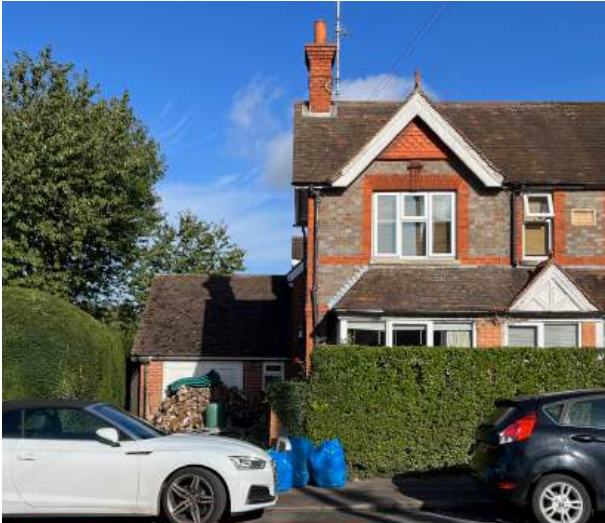
South elevation view from Victoria Road
